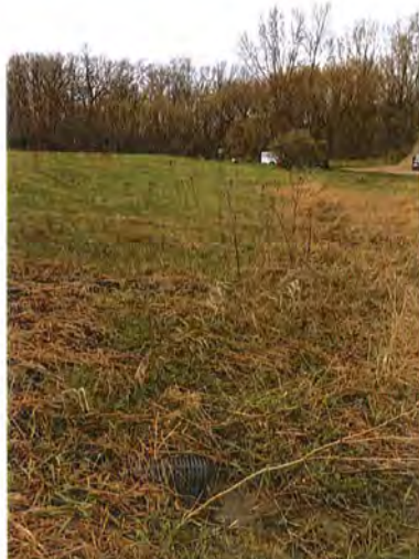
Figure 3: Drainage Pipe, located at South West corner
