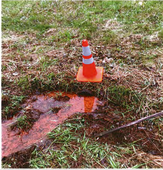
Figure 1: Drainage Pipe, located at SE corner.
