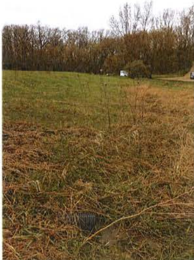
Figure 3: Drainage Pipe, located at South West corner
