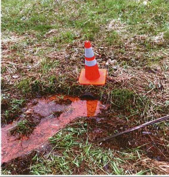
Figure 1: Drainage Pipe, located at SE corner.
