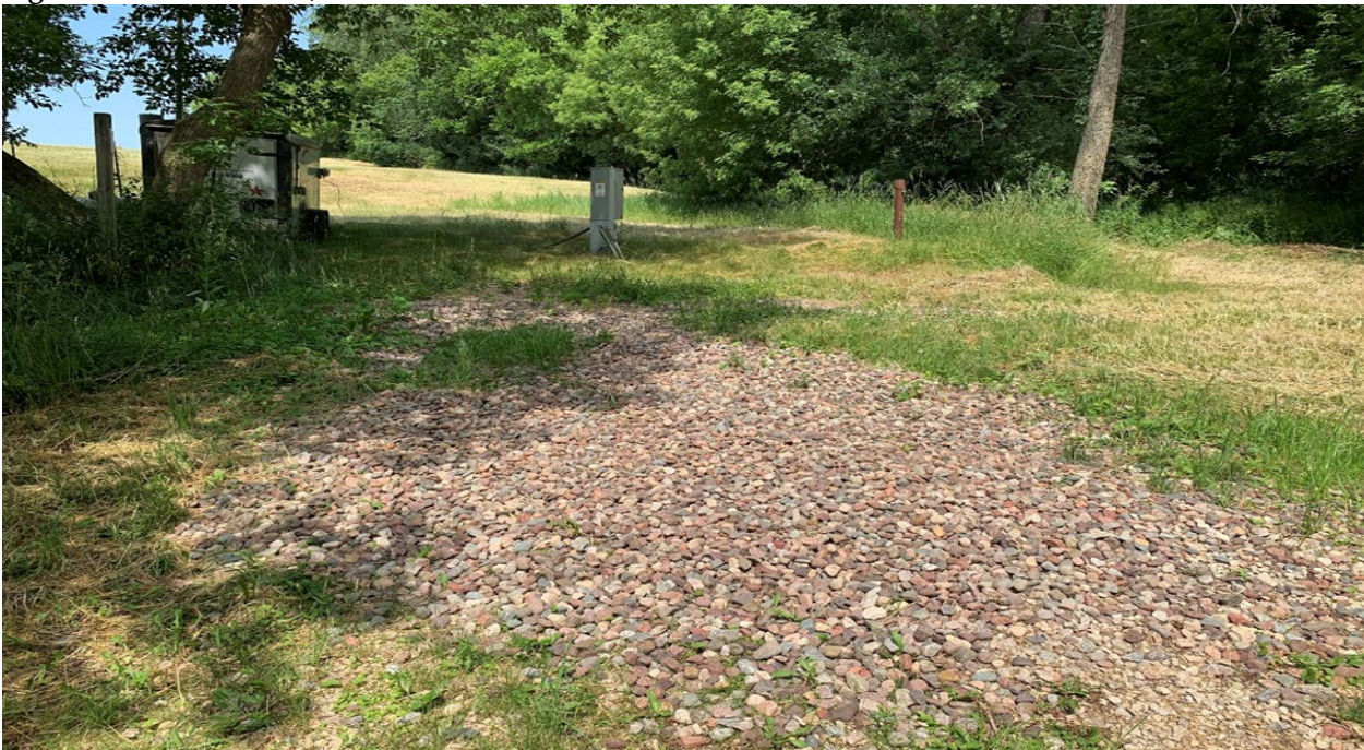
Figure 2: Outfall stone from contoured drainage ditch at SE corner.
