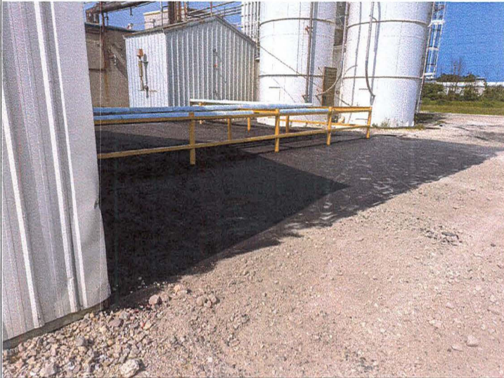
Title: Asphalt cap over former excavation area.
