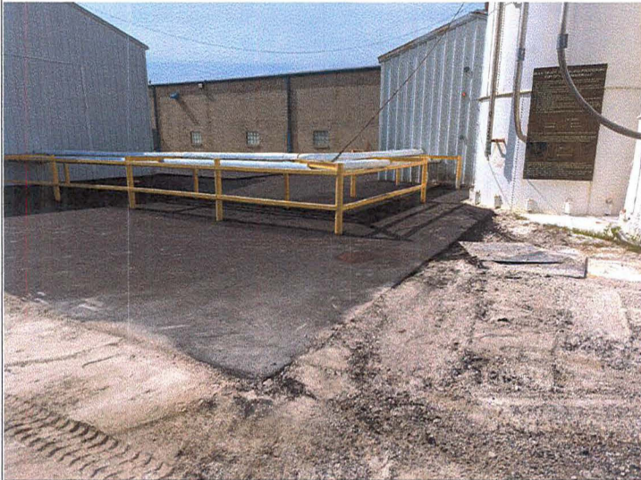
Title: Asphalt cap between plasticizer building and silos.
