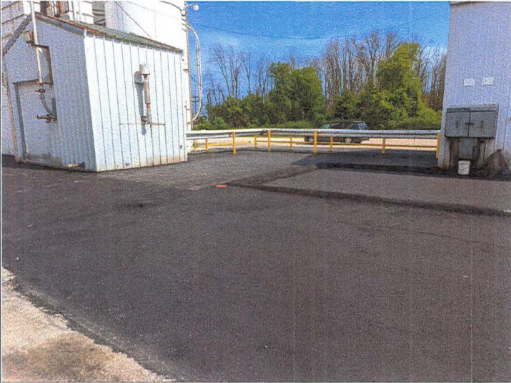
Title: Asphalt cap in place between plasticizer building and shed/silos.
