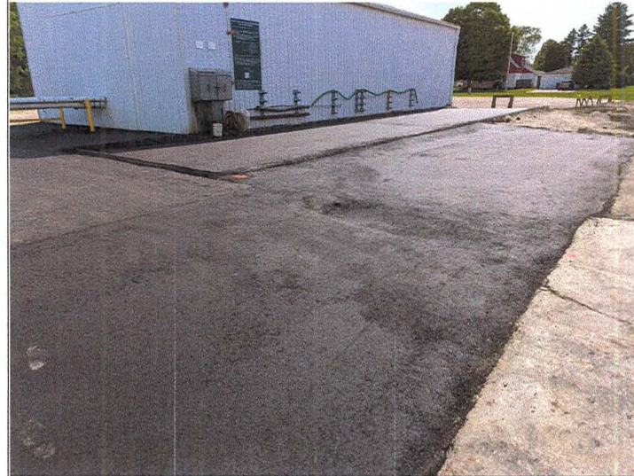
Title: Asphalt cap north of plasticizer building.
