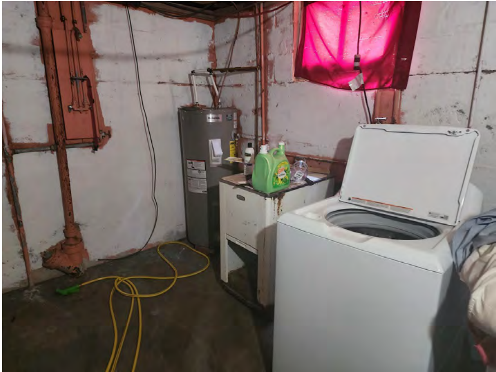
Water heater and sewer pipe
