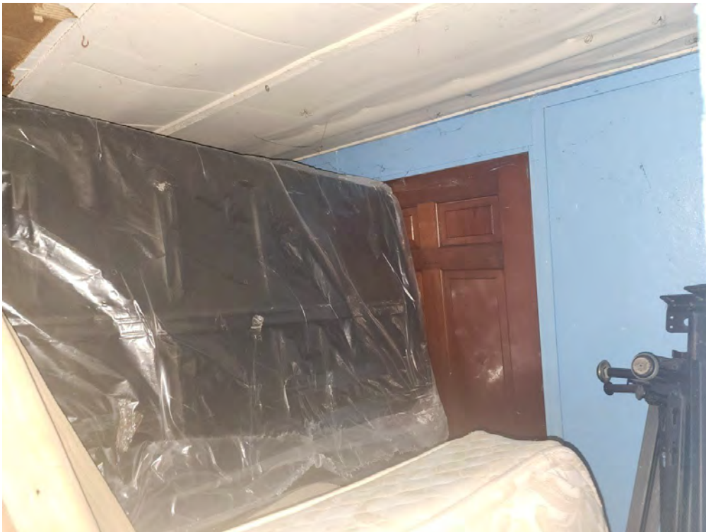
Under porch storage, door not accessible.
