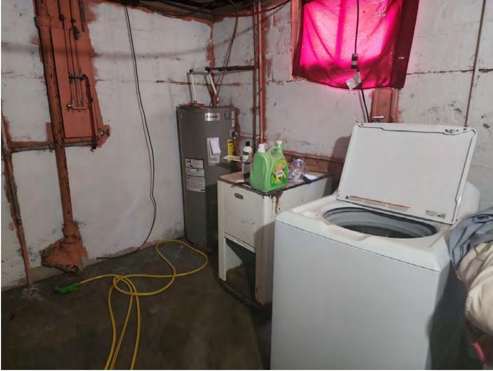
Water heater and sewer pipe
