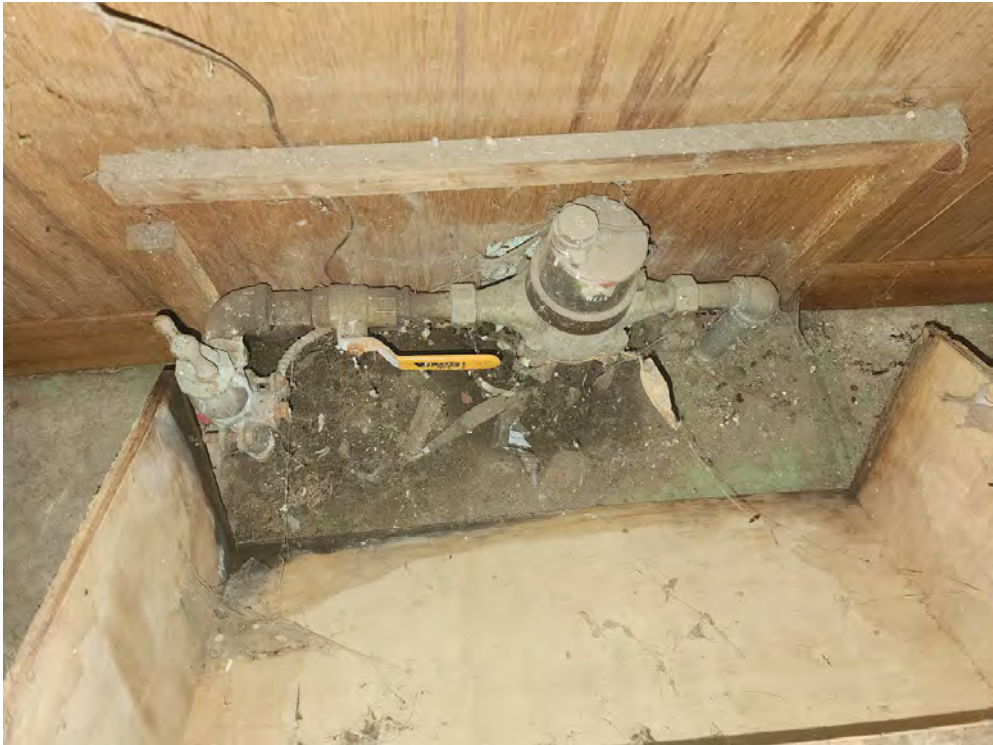
Pipe by stairs
