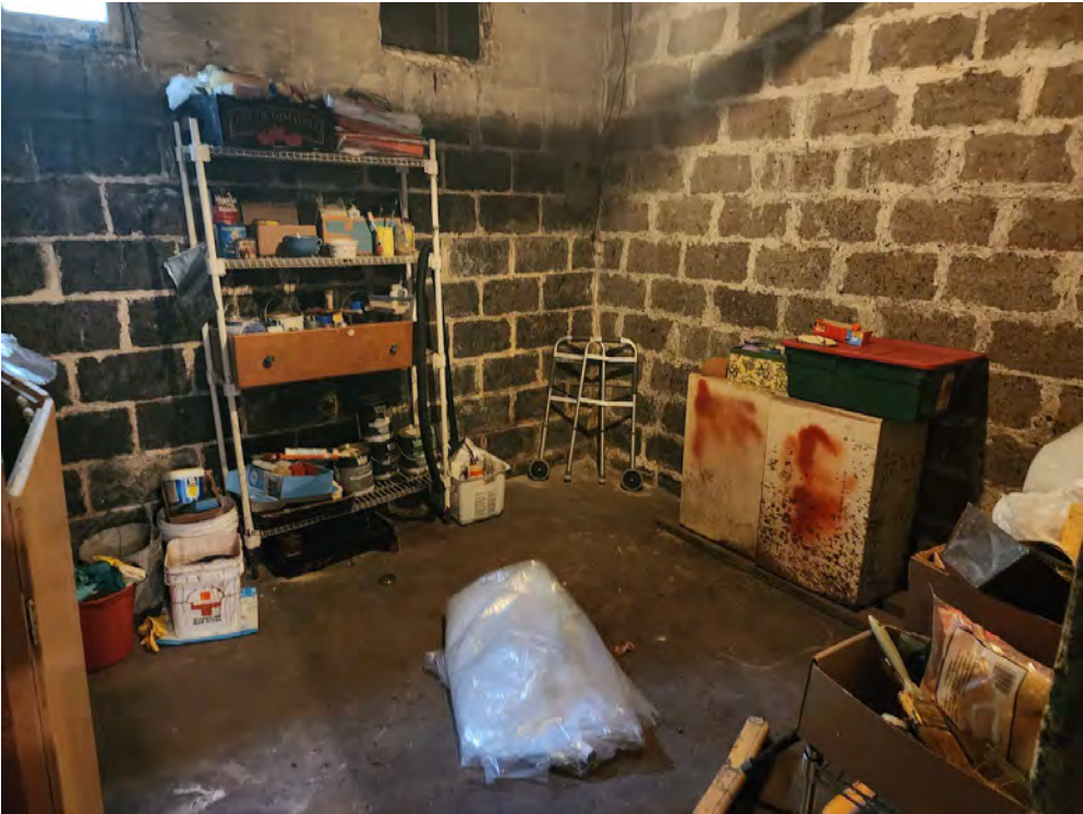
Coal Chute room
