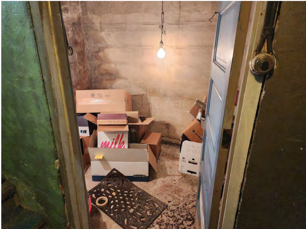
Former dark room
