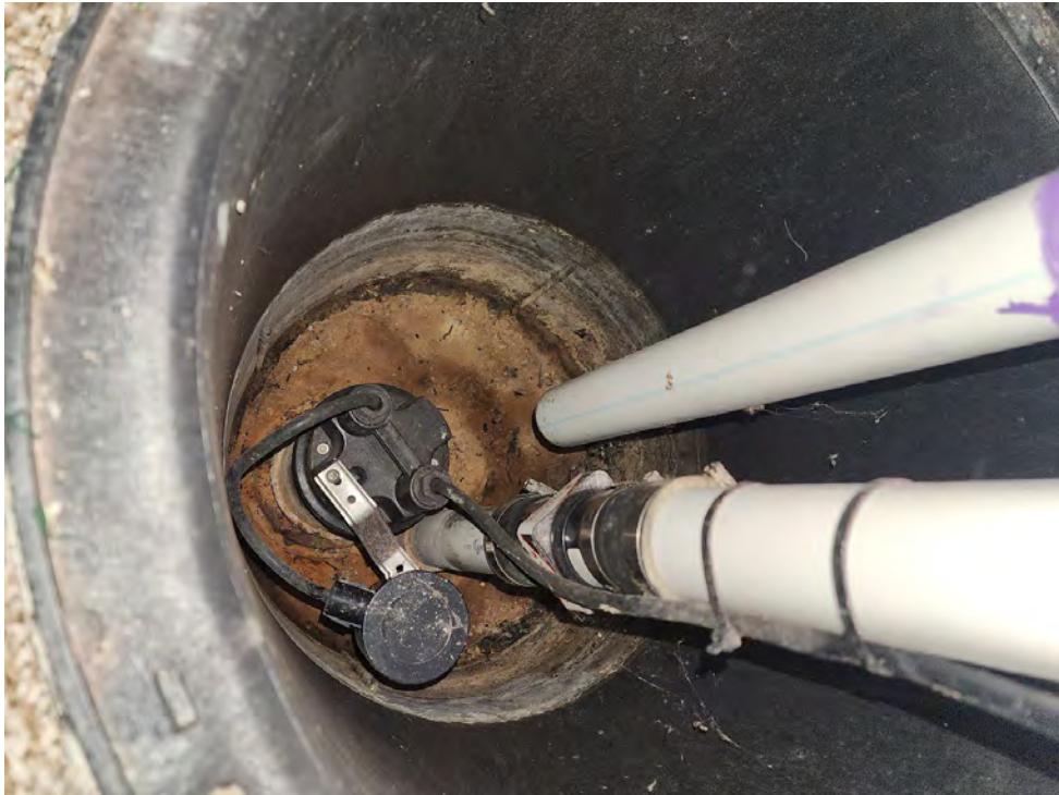
Inside sump pit
