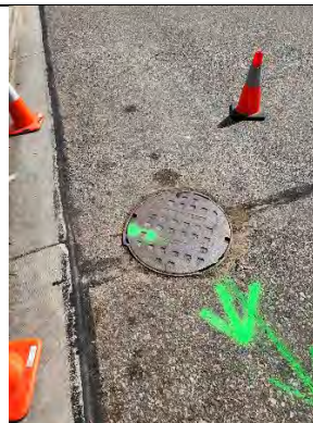
Photo 3: Manhole as left
