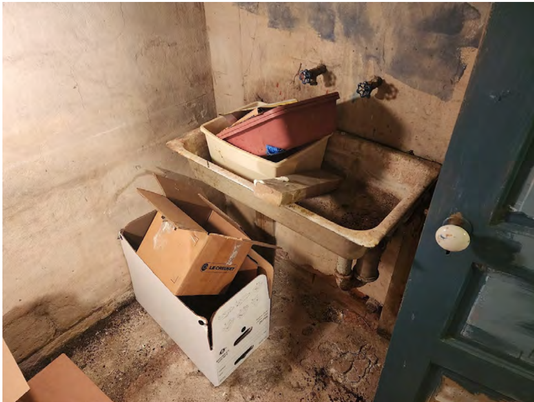
Dark room sink
