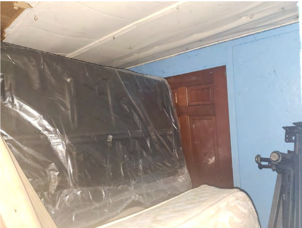
Under porch storage, door not accessible.
