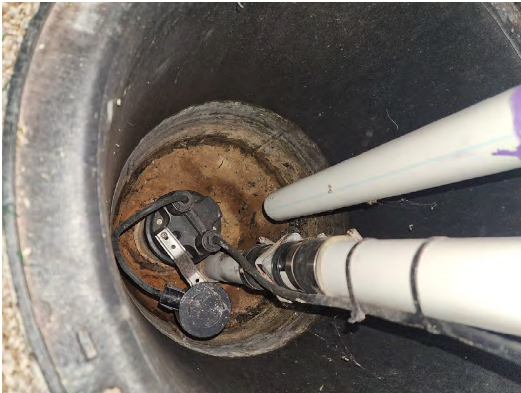
Inside sump pit
