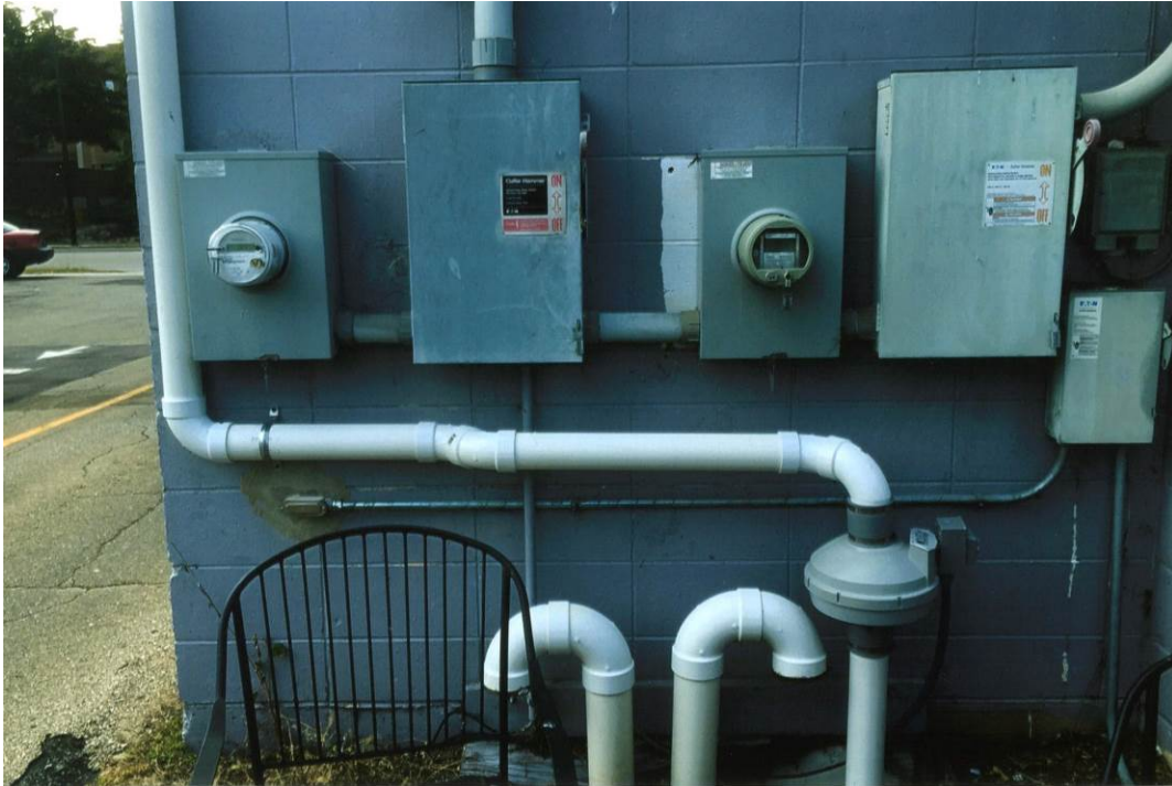
Photo 5: Looking west at east side of 3918 Monona Drive VMS fan and discharge piping.
