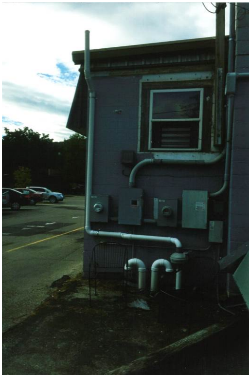
Photo 5: Looking west at east side of 3918 Monona Drive VMS fan and discharge piping.
