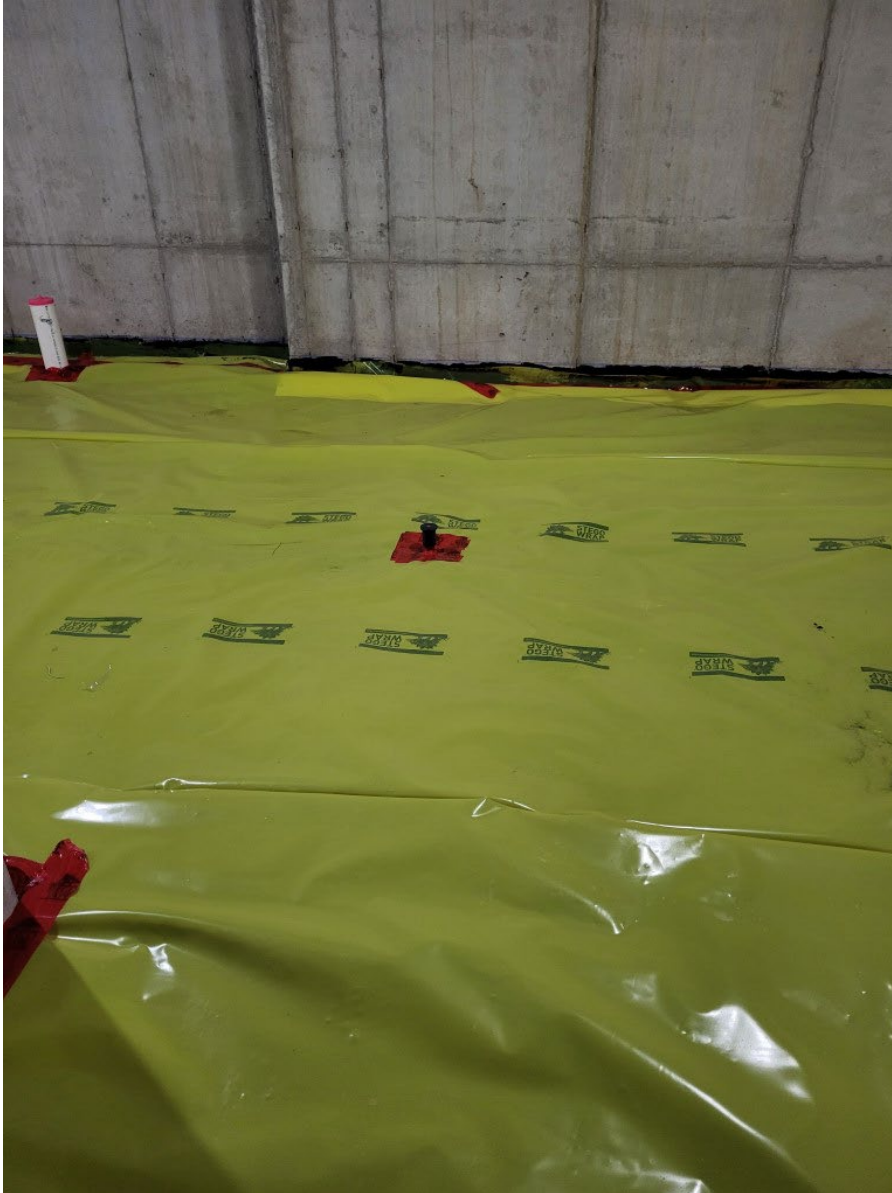
Photo 6: VP-3 installed and sealed into vapor barrier (10/5/2023; 15:36).
