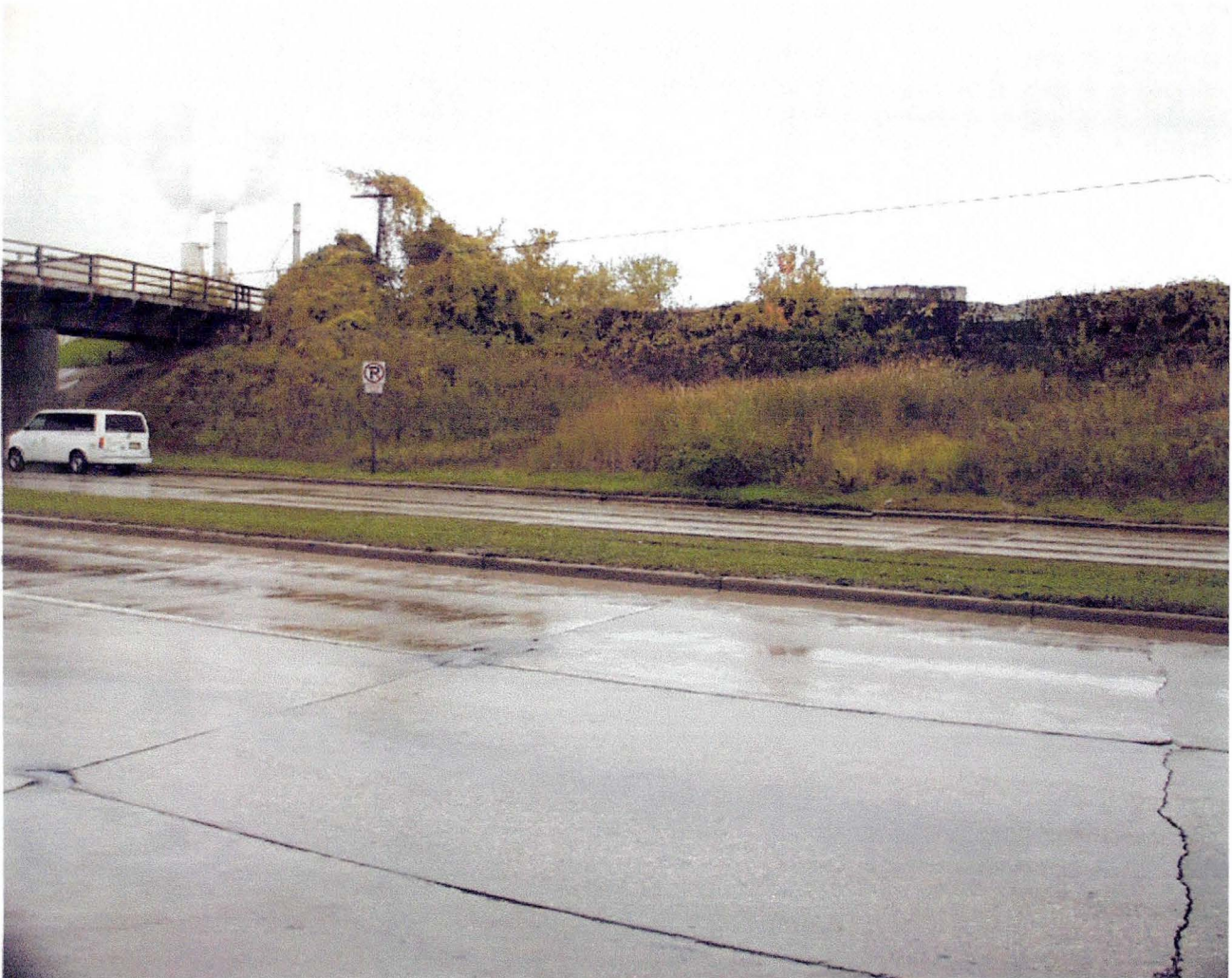
West Silver Spring Drive, just east of North 124th Street between the railroad overpasses, looking Northwesterly. The water source is located about 30 feet from the curb directly behind the "No Parking" sign.
