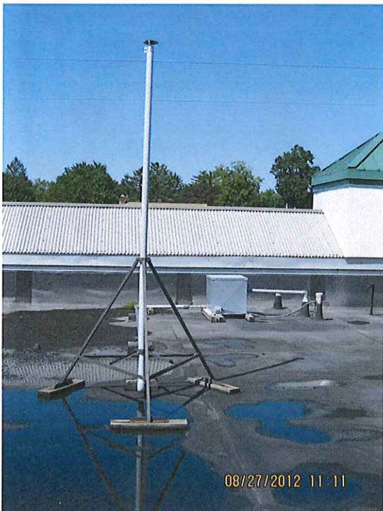
Vent pipe stack on roof.
