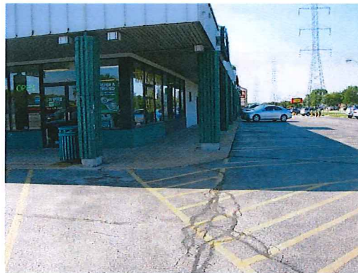
Exterior facing South
