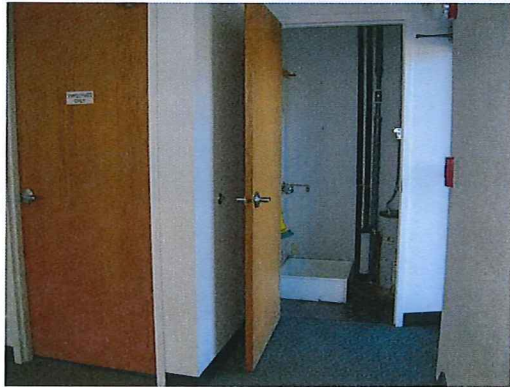
Passive vent room at distance
