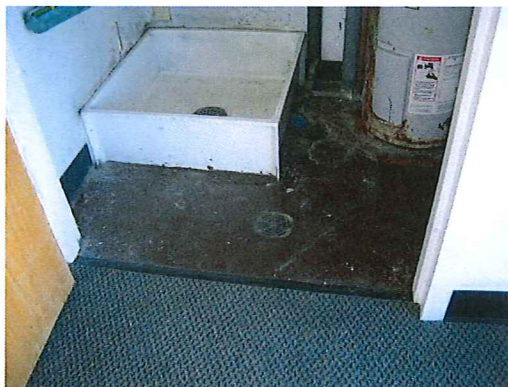
Passive vent room w/exposed epoxy floor
