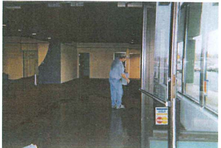
2. Applying silica sand to ECO-POXI floor.
