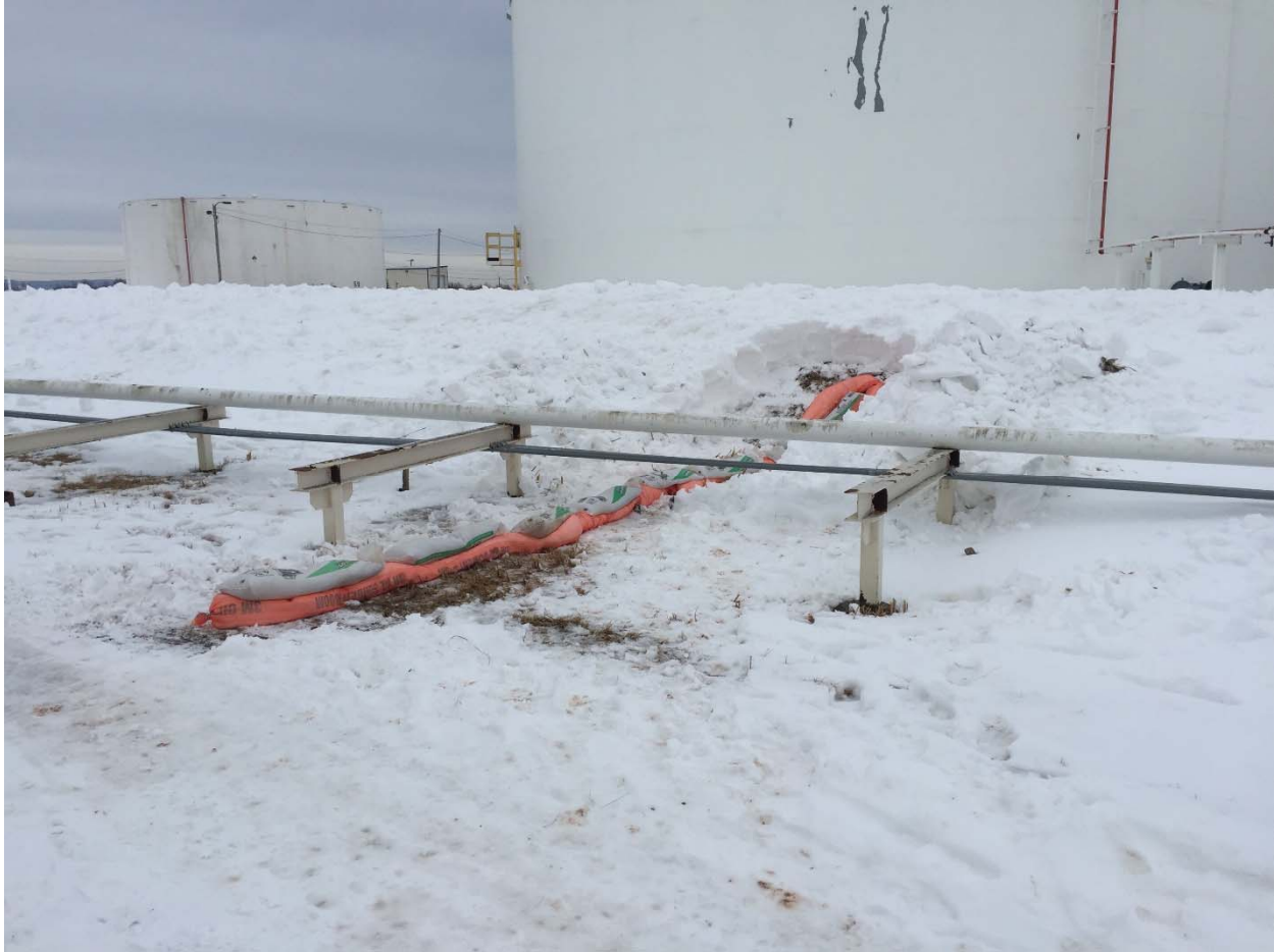
Photo 6: Looking northeast at the absorbent boom deployed along the eastern edge of the tank containment dike. This was placed upgradient (north) of the dike drain valve pooling location as a precaution.
