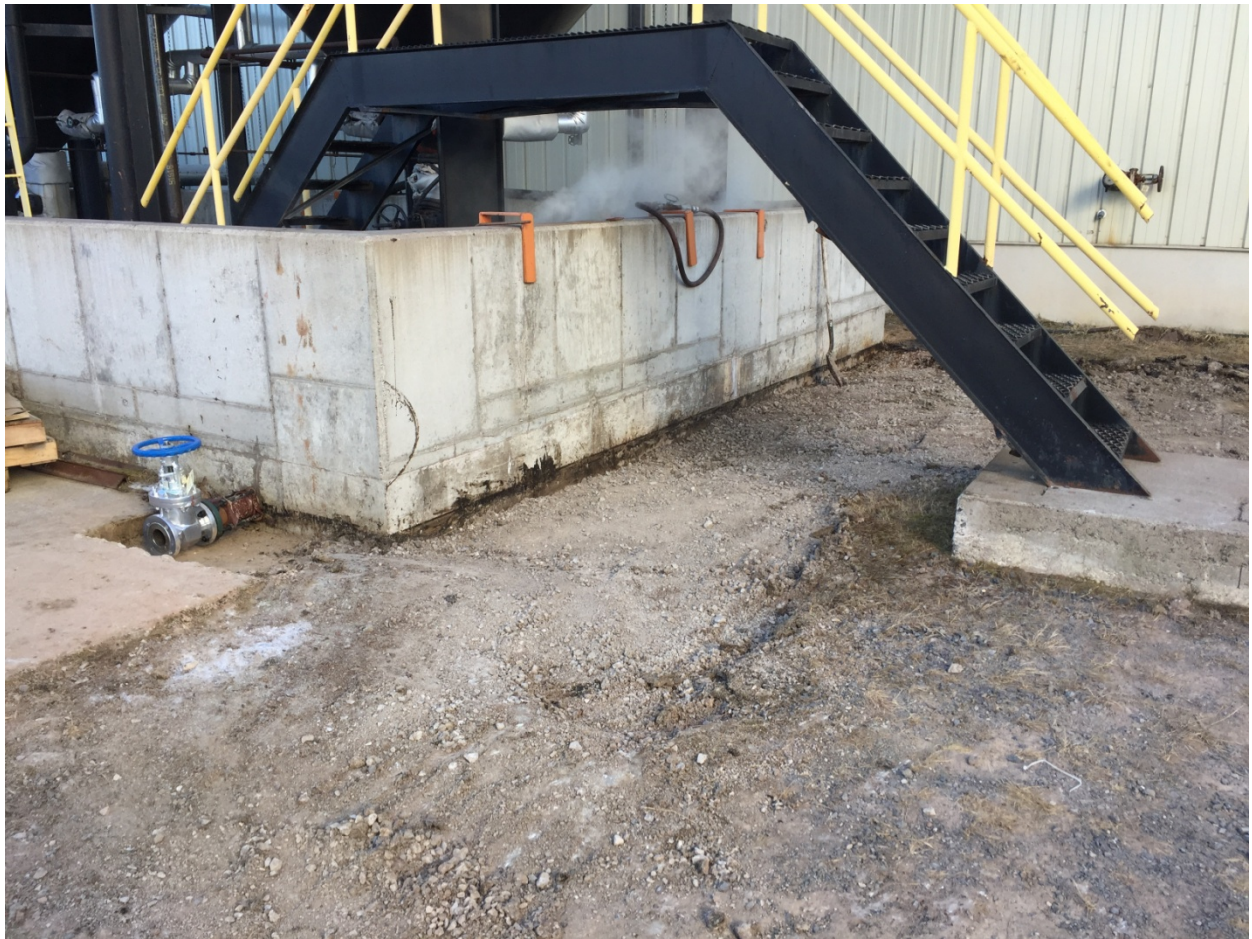
Photo 6: Looking southeast at the excavation.
