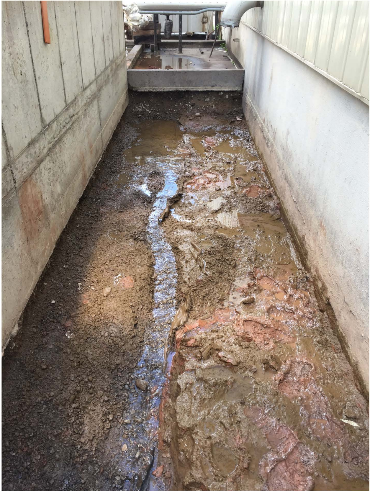
Photo 8: Looking east at the excavation.
