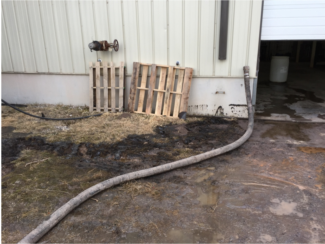
Photo 5: Looking south at the release area.
