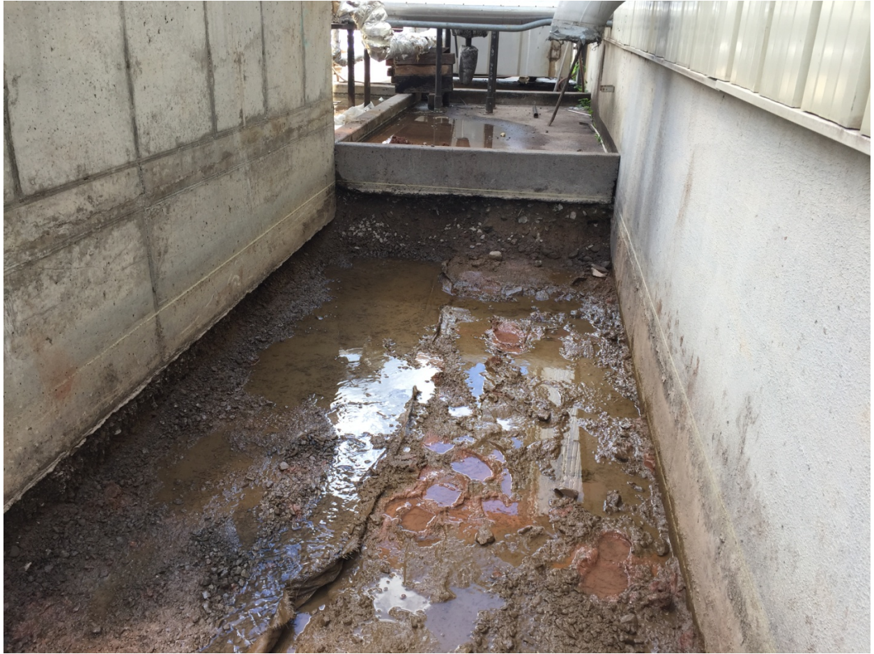
Photo 7: Looking east at the excavation.
