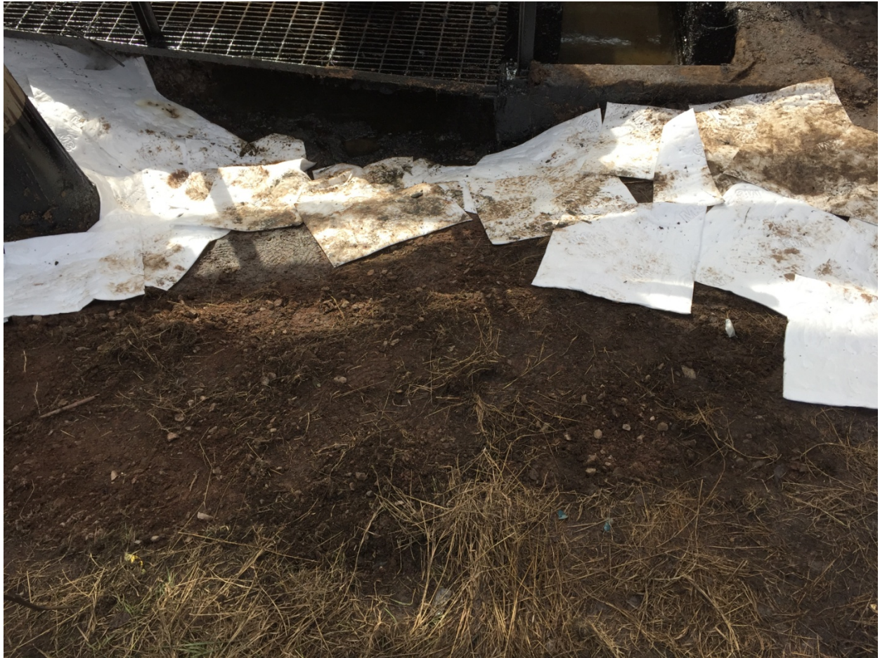
Photo 9: Looking south at the scraped and exposed visually clean soil. The grass line marks the northern extent of the release.
