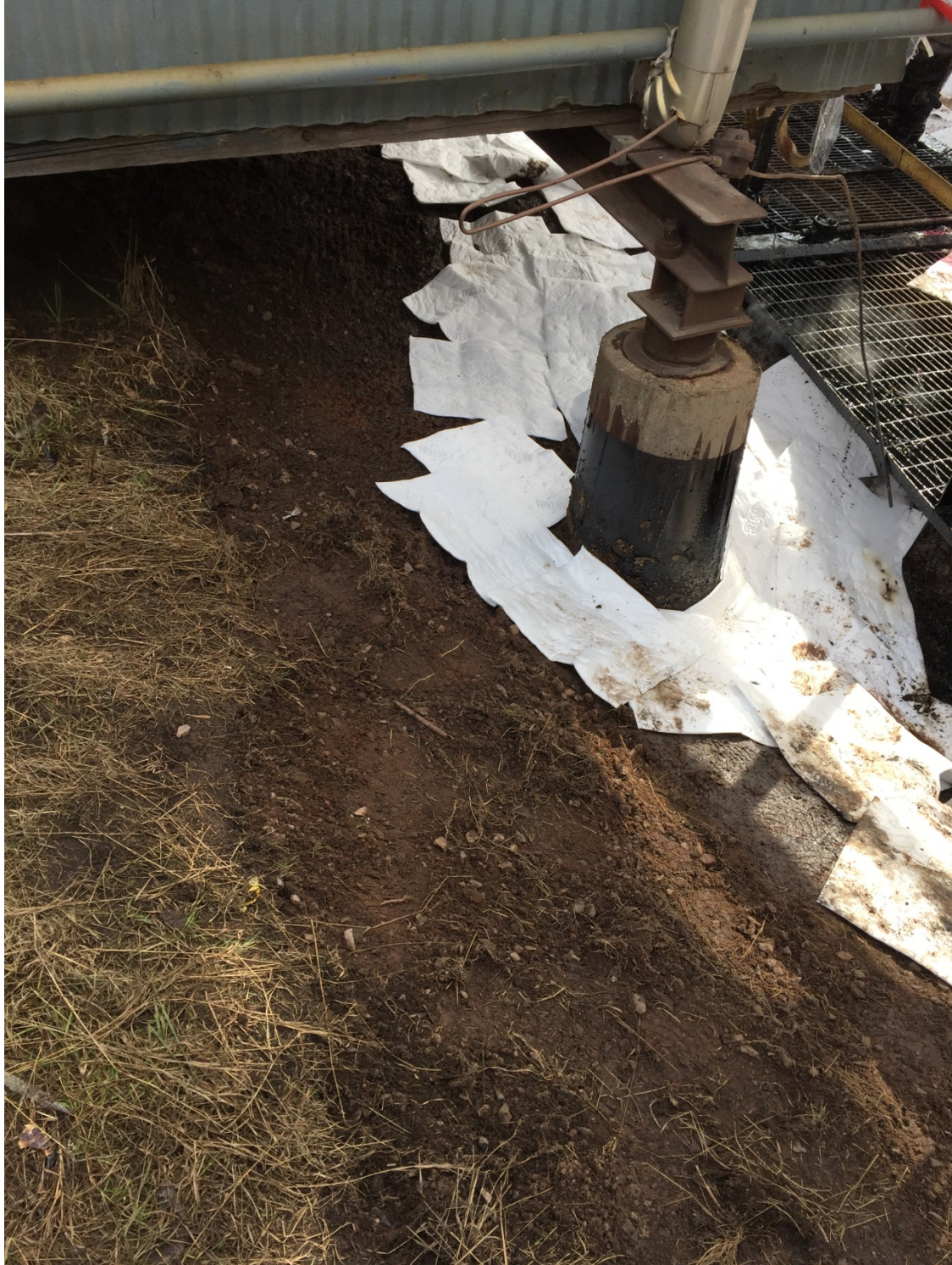
Photo 8: Looking southeast at the scraped and exposed visually clean soil. The grass line marks the extent of the release.
