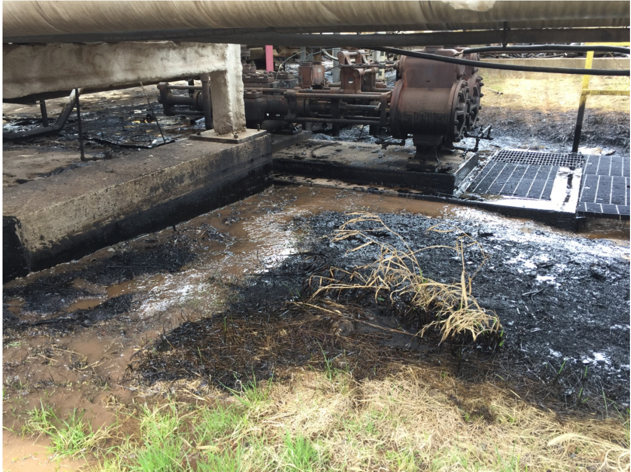
Photo 2: Looking north at the release site. The water seen entering the release site is runoff from the road located uphill and south of the release site. A sand dam and absorbent boom were placed at the edge of the road to prevent further water from entering the site. This can be seen in Photo 6.
