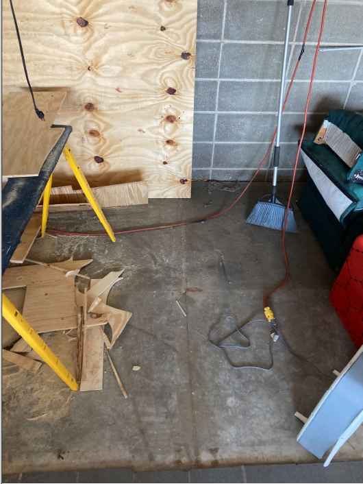
Title: Village Clean - View of Indoor Soil Cap building floor slab, no repairs needed
