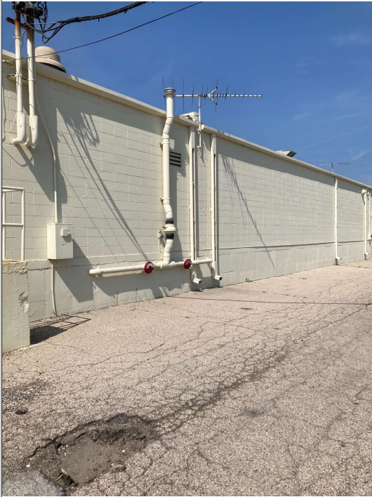
Title: Village Clean - View of VMS and Soil Cap, VMS operating successfully, soil cap needs repair
