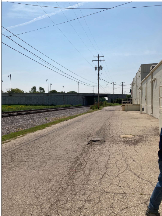
Title: Village Clean - View of Alley Soil Cap, soil cap needs repair
