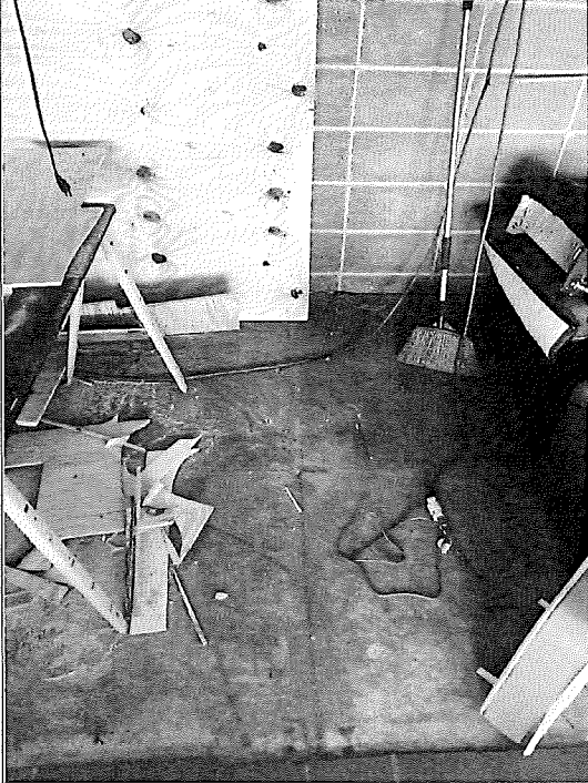
Title: Village Clean - View of Indoor Soil Cap building floor slab, no repairs needed
