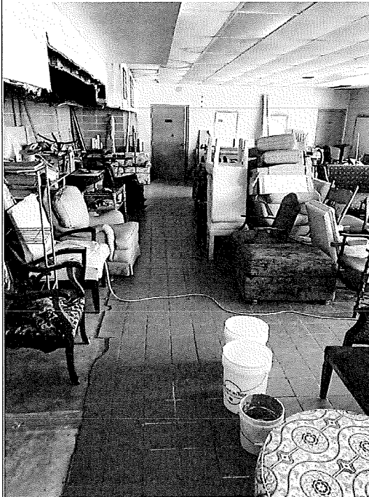
Title: Village Clean - View of Indoor Soil Cap building floor slab and tiles, no repairs needed
