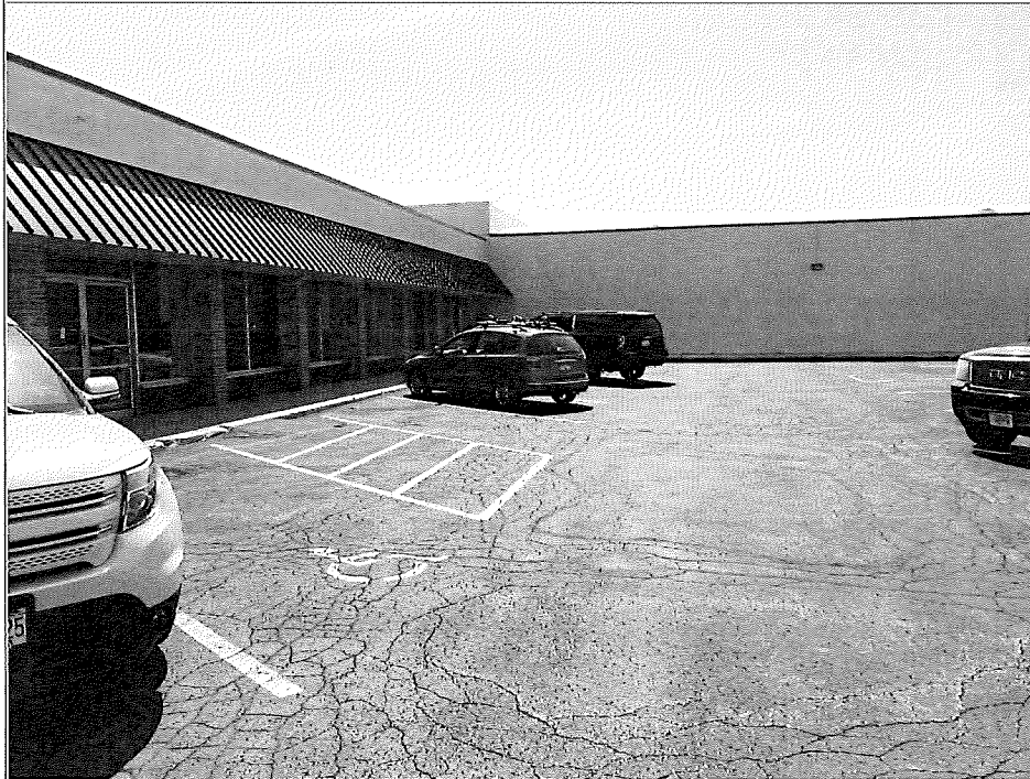
Title: Village Clean - View of Parking Lot Soil Cap, soil cap needs repair
