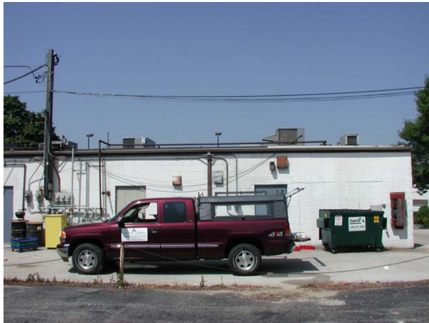
One-Hour Martinizing - N. Teutonia Ave. North view of asphalt cap
