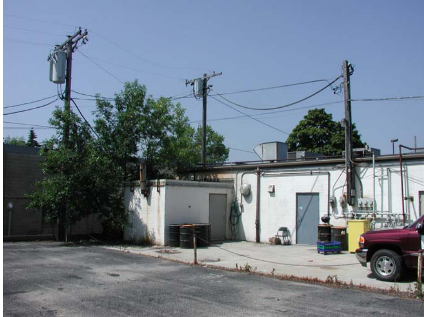
One-Hour Martinizing - N. Teutonia Ave. South view of asphalt cap
