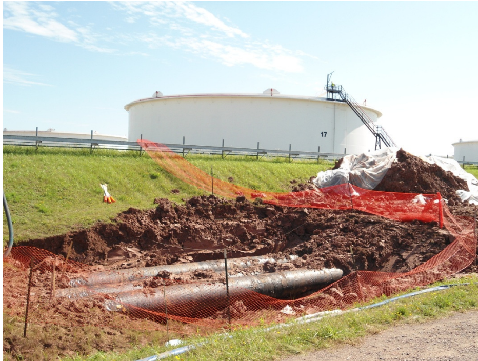
Picture 1: Tank 16-17 excavation on August 15, 2011.
