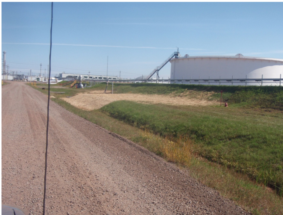
Picture 2: Backfilled and restored excavation on September 28, 2011.
