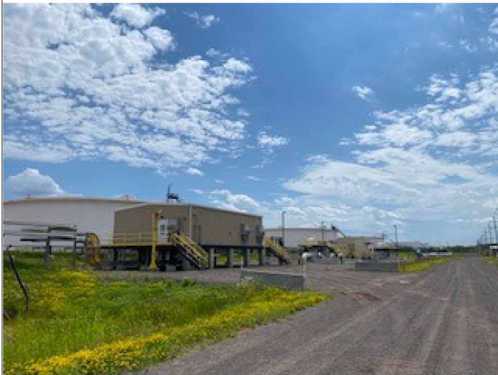
Title: Infrastructure near middle of Nemadji Corridor. Photo taken facing southwest on 7/18/2022.
