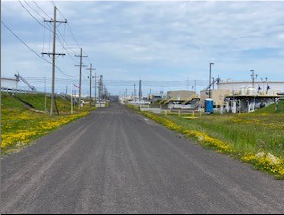
Title: Southwest end of Nemadji Corridor. Photo taken facing northeast on 7/18/2022.
