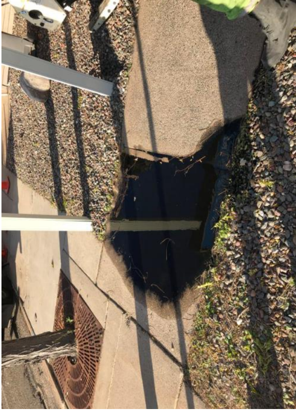
Daylighted formation water and carbon slurry
