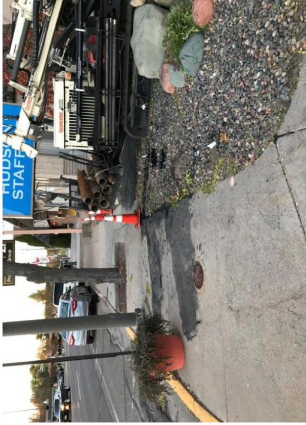
Area of daylighted formation water and carbon slurry near AAMW7
