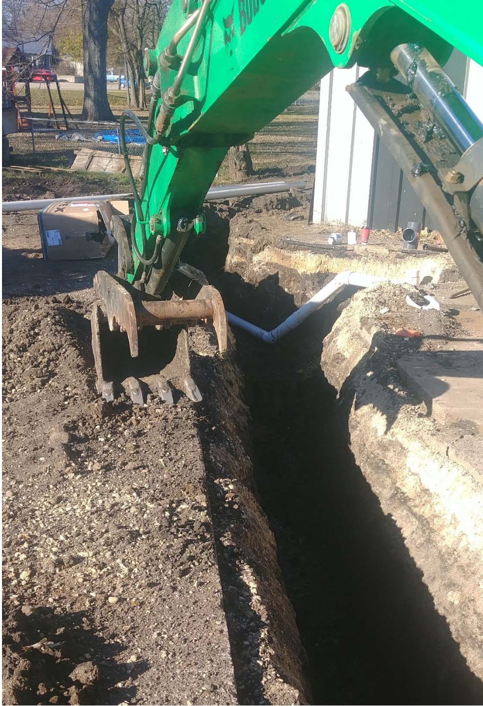
Trenches on south side of building, facing northwest.
