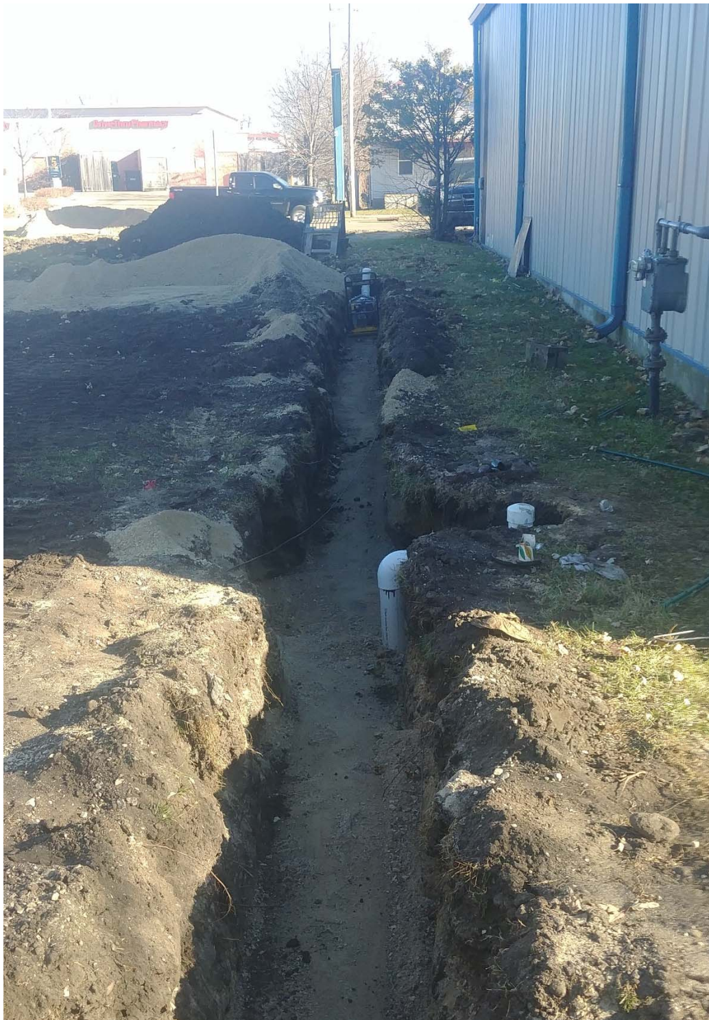
Trench to SVE-4 and SVE-5 during backfilling, facing east.
