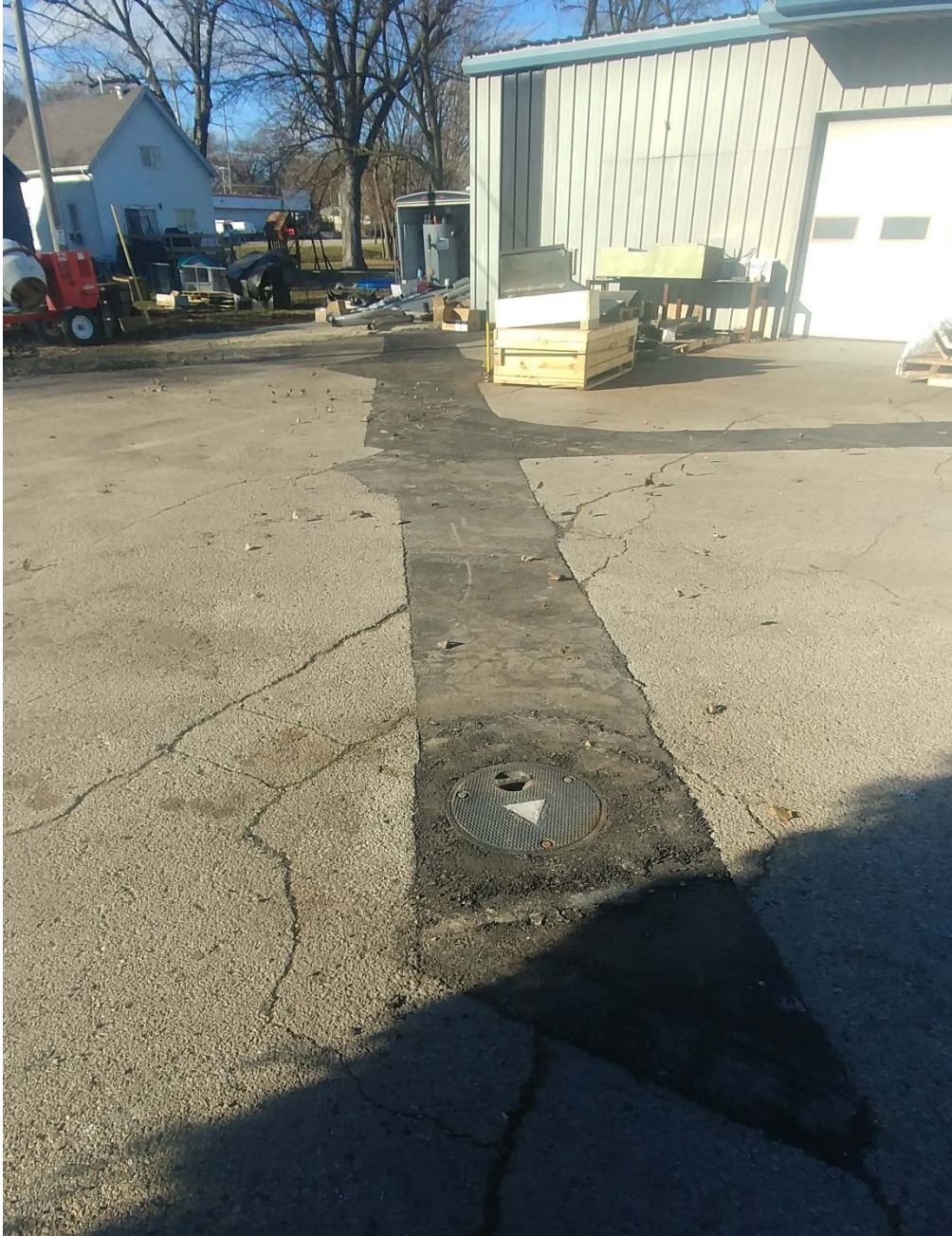
Trench from SVE-3 with asphalt patch, facing northwest.
