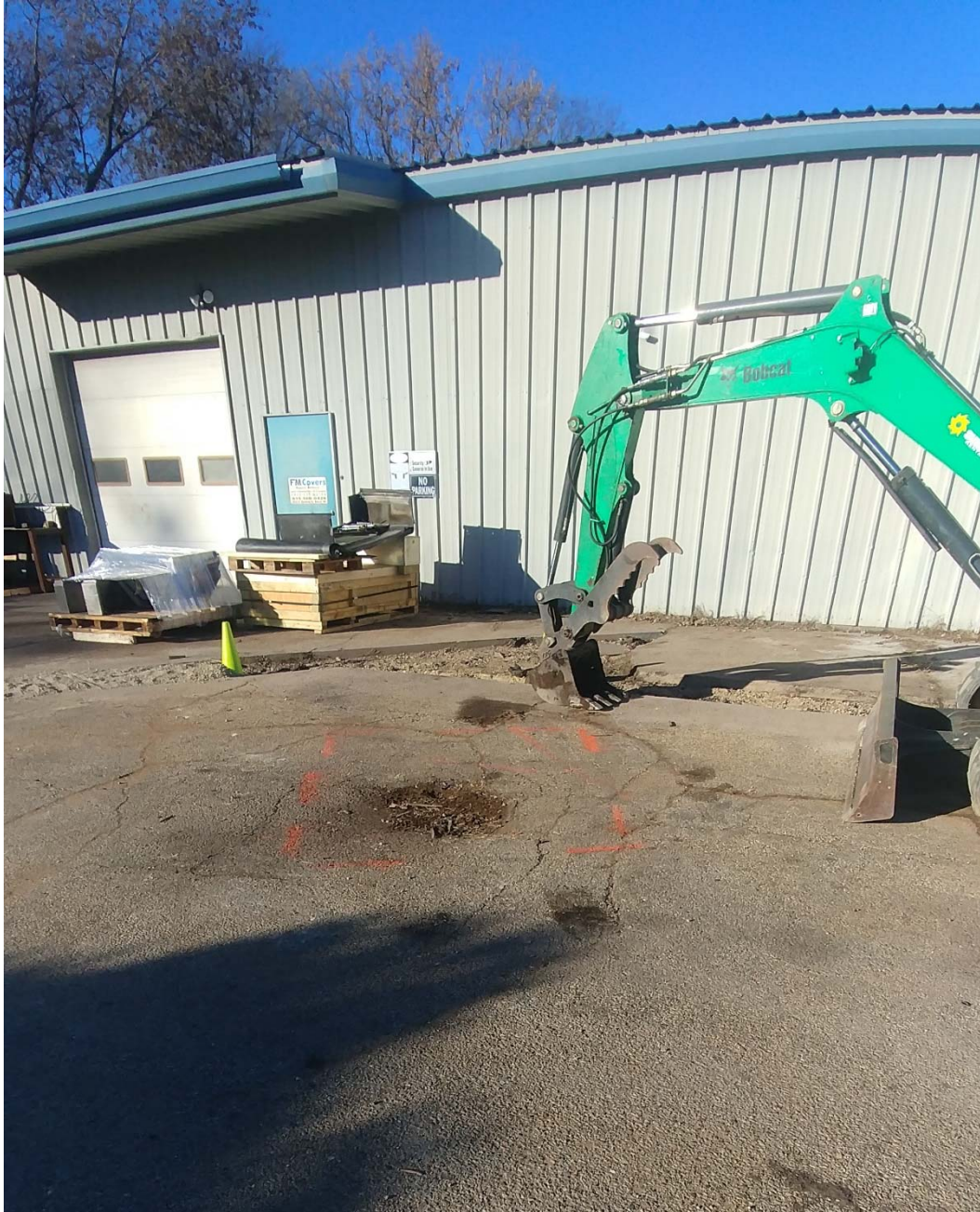
Beginning trench excavation on south side of building, facing northwest.
