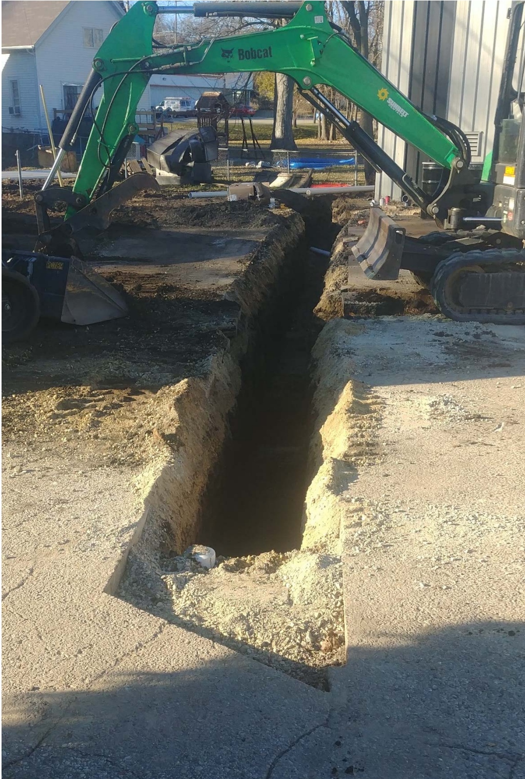
SVE-3 and trench toward equipment trailer, facing northwest.
