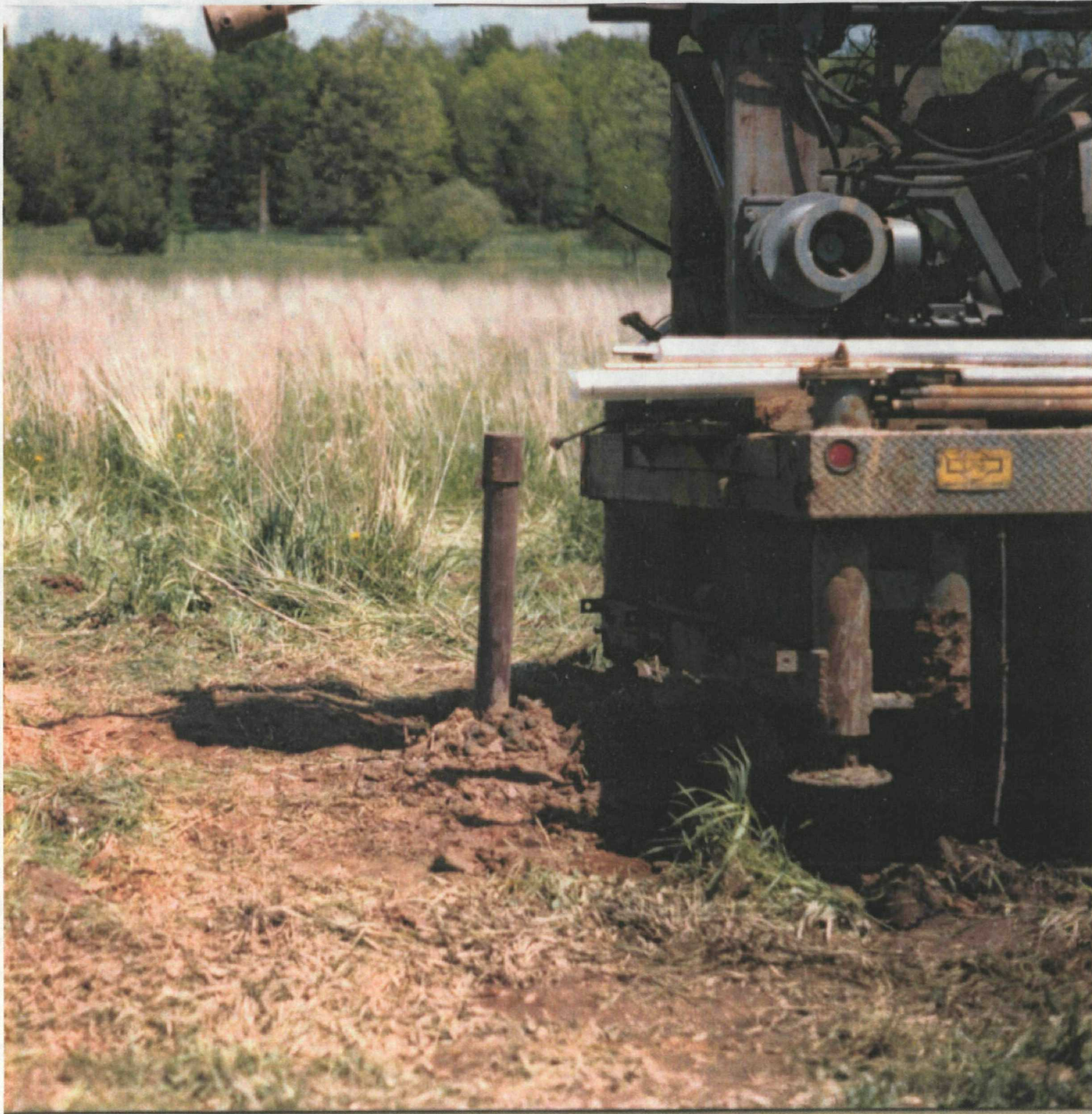
PHOTO 6 6/6/2002 Photo taken by John Grump DRILLING MW-15A APPENDIX A
