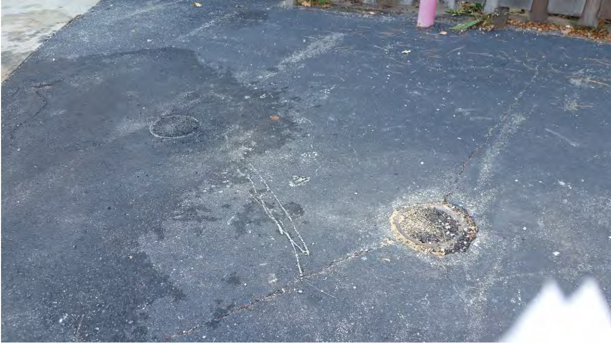
Photo 7: Abandoned monitoring wells MW-8 and MW-8P
