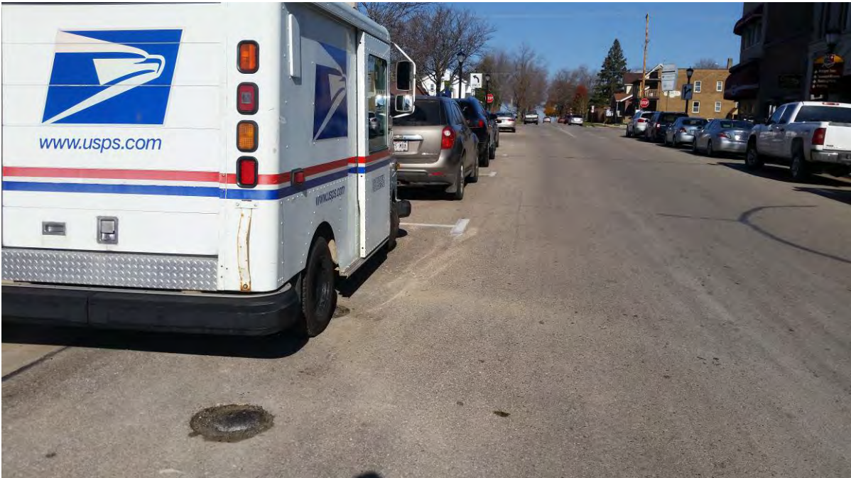
Photo 10: Abandoned monitoring wells MW-11 and MW-11P (MW-11 in front of truck tire)
