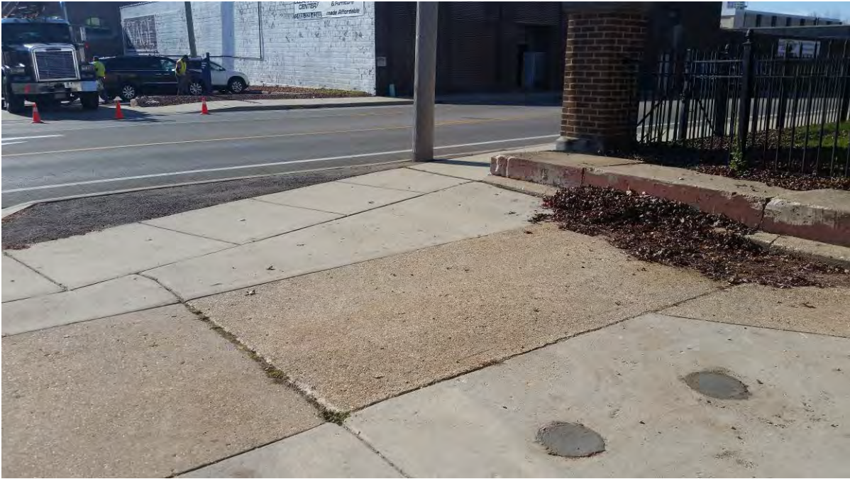
Photo 1: Abandoned monitoring well MW-1 and SVE well SVE-1
