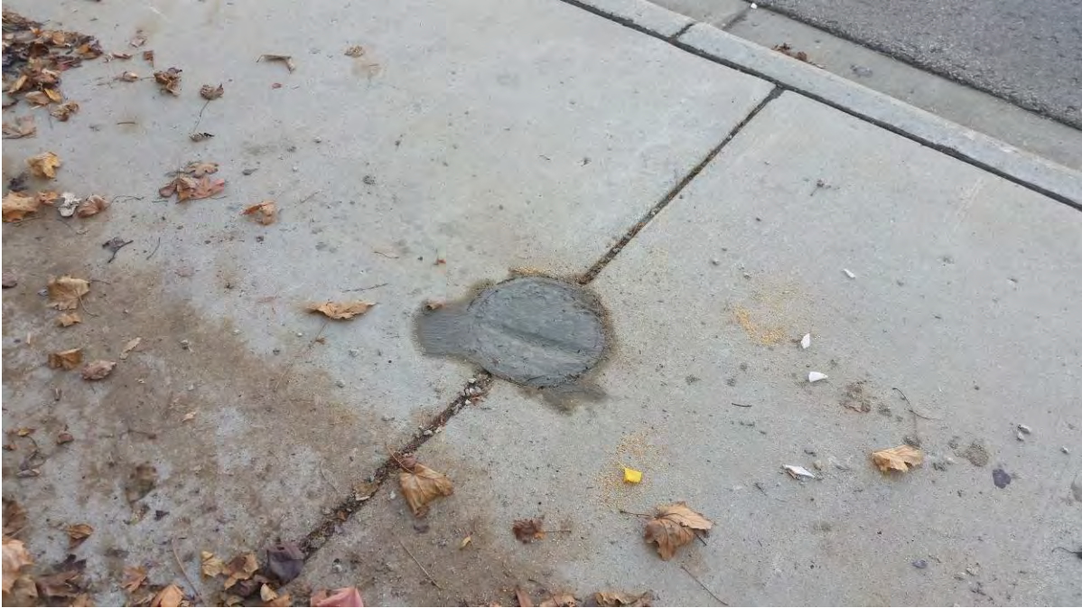
Photo 9: Abandoned monitoring Well MW-10
