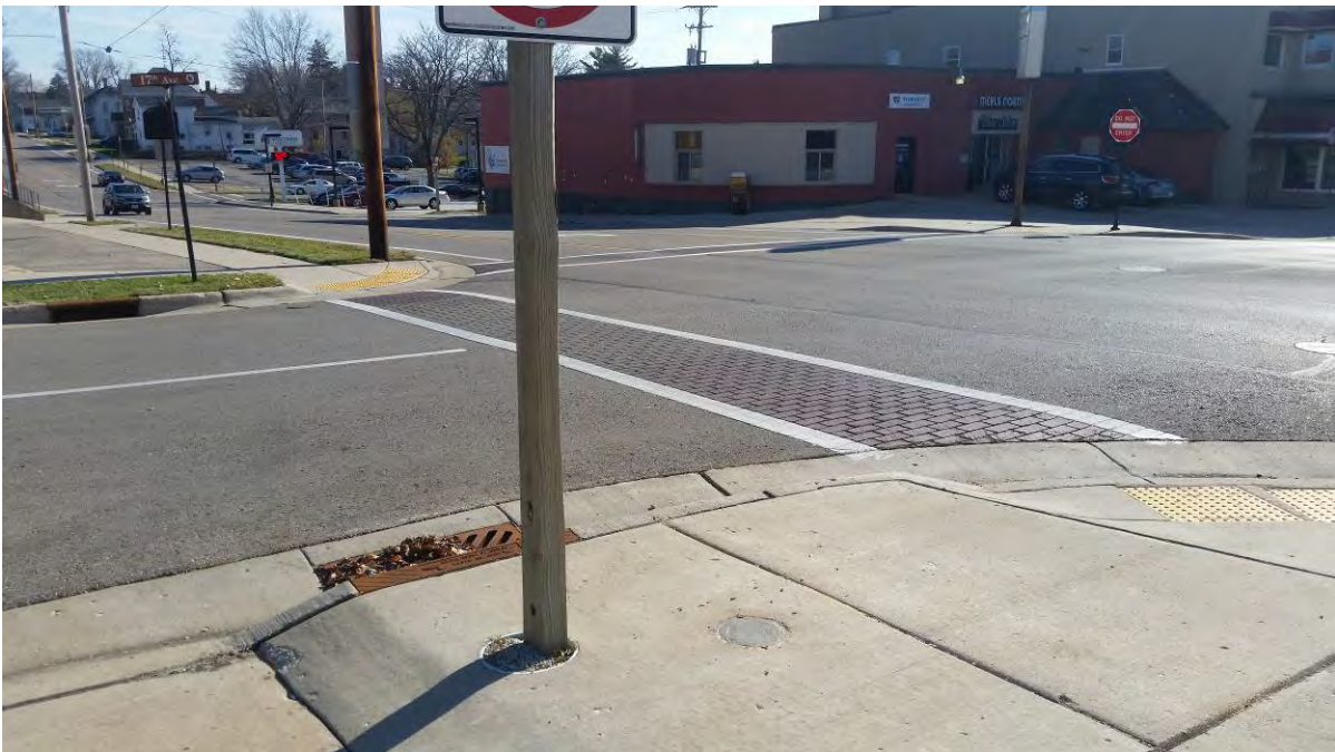
Photo 12: Abandoned monitoring well CMW-8
