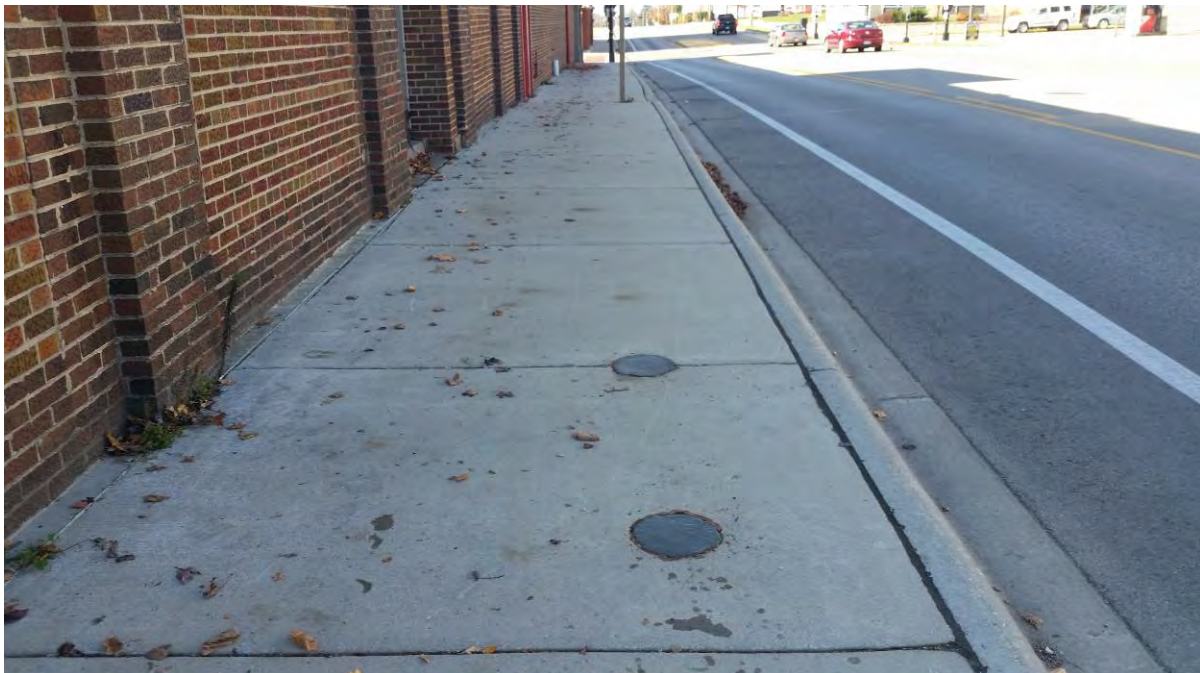
Photo 6: Abandoned monitoring wells MW-7 and MW-7P
