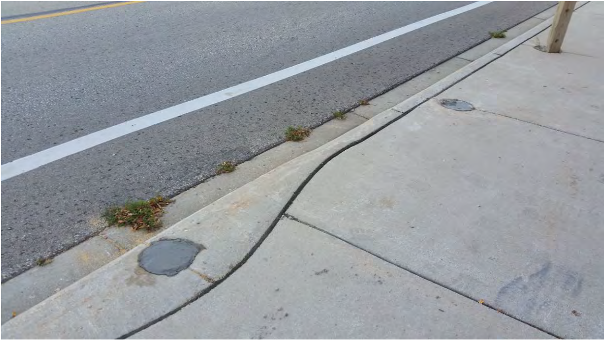
Photo 11: Abandoned monitoring wells CPZ2 and CMW6
