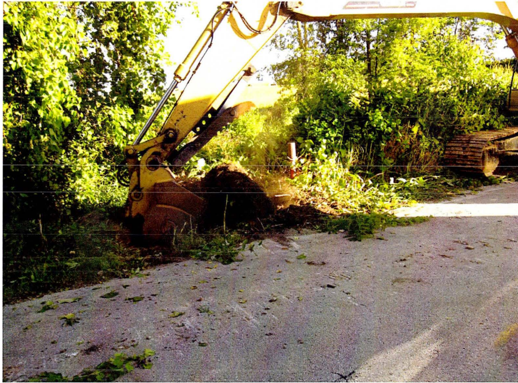
Photo 1 Start of excavation around MW-3
