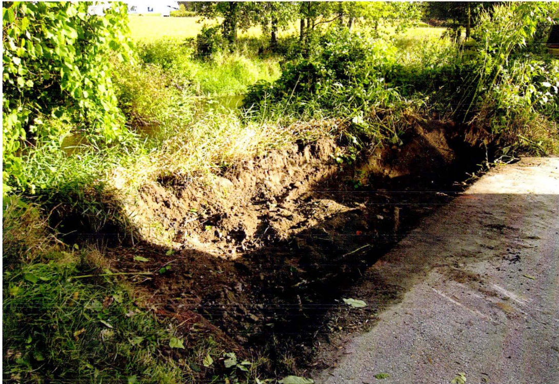
Photo 2 Excavated area around former MW-3
