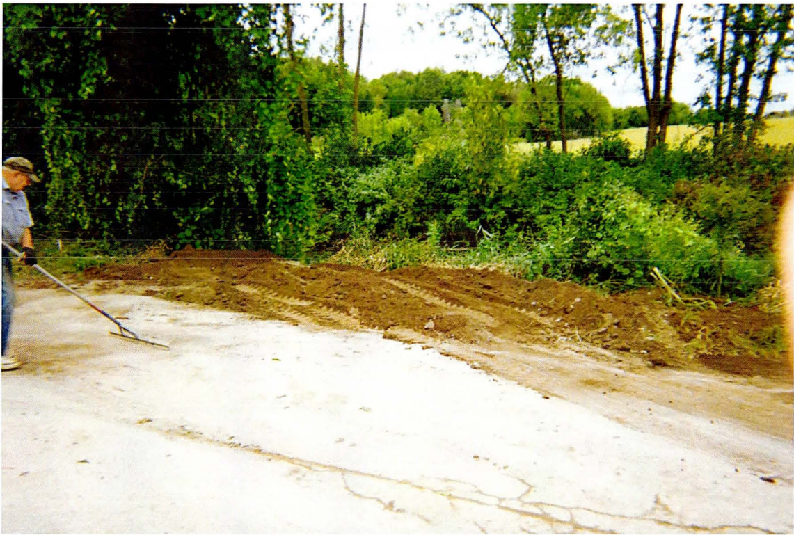
Photo 5 Top-soil placement near MW-3
