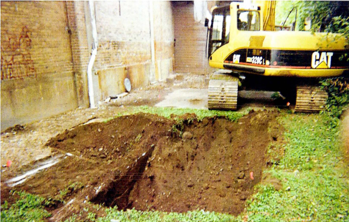
Photo 4 Excavation starting near SB-4.
