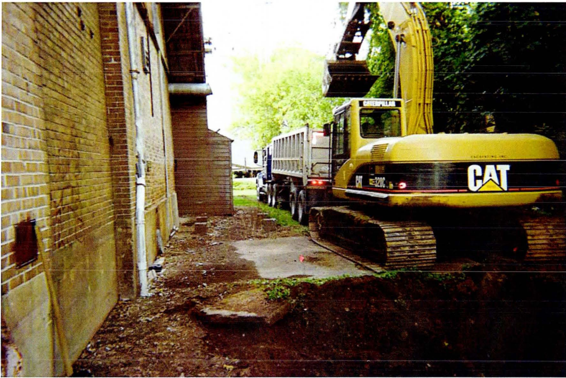
Photo 3 Excavation and loading of soils near SB-4
