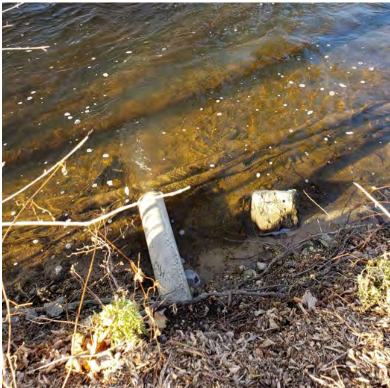
Photo 2: North Outfall photo taken by Ramboll on December 10, 2020
