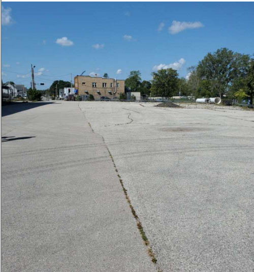
Title: Utility work asphalt replaced (left side), Asphalt cap (right side).
