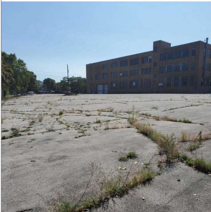
Title: Asphalt cap area to be maintained in area where PAHs were documented in soil, looking southeast.
