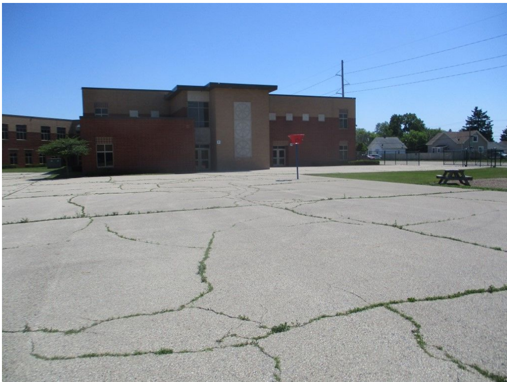
ASPHALT PLAY AREA & SCHOOL BUILDING, FACING SOUTH-SOUTHWEST
