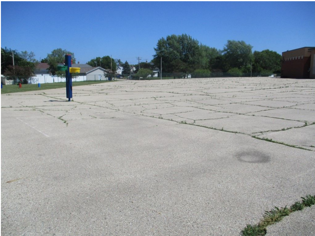
ASPHALT PLAY AREA FACING SOUTHEAST
