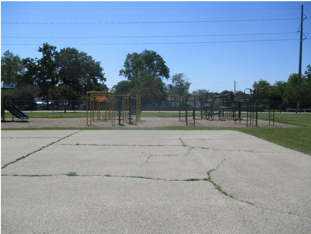
ASPHALT & PLAY AREA, FACING WEST
