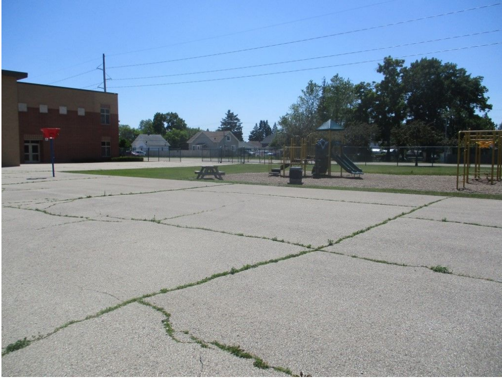
ASPHALT & PLAY AREA, FACING SOUTHWEST
