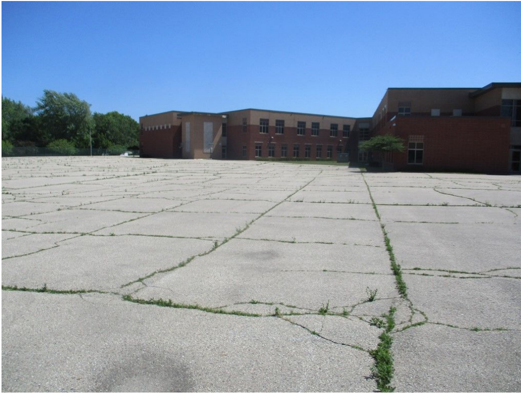
ASPHALT PLAY AREA & SCHOOL BUILDING, FACING SOUTH
