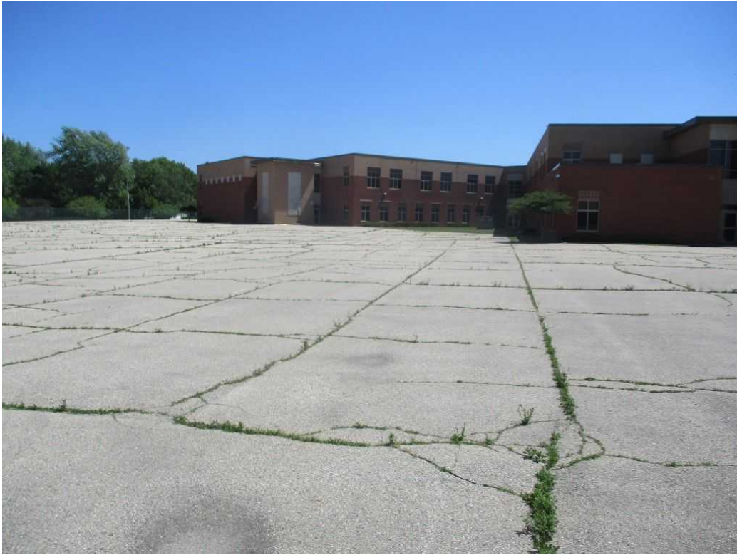
ASPHALT PLAY AREA & SCHOOL BUILDING, FACING SOUTH
