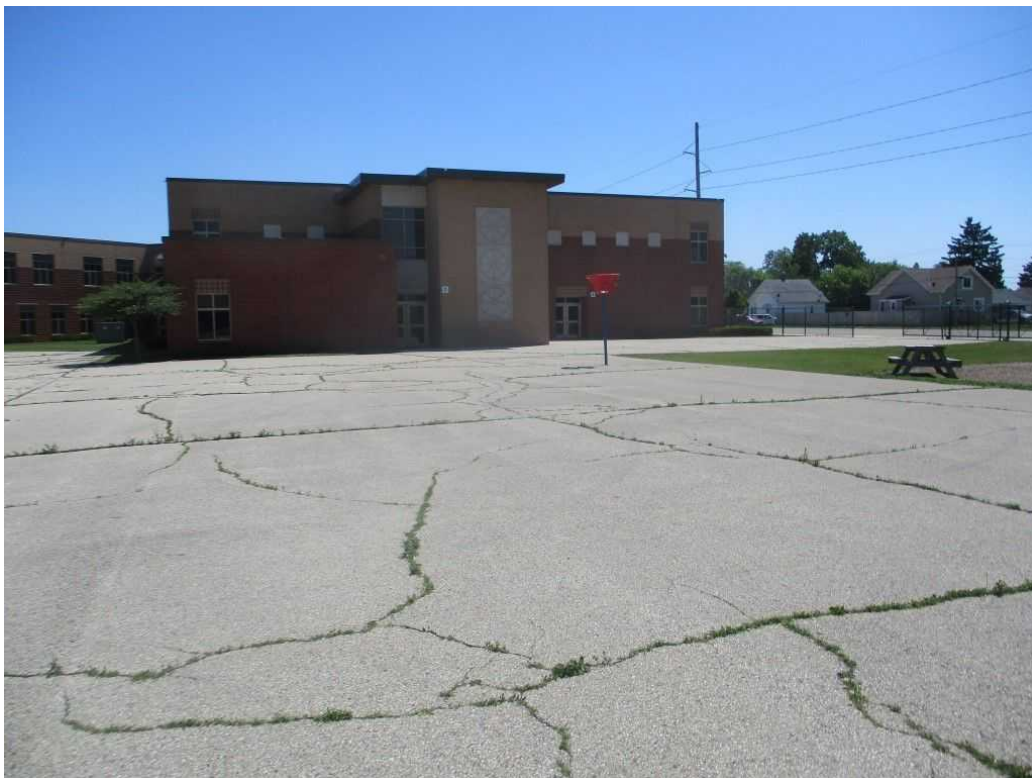
ASPHALT PLAY AREA & SCHOOL BUILDING, FACING SOUTH-SOUTHWEST
