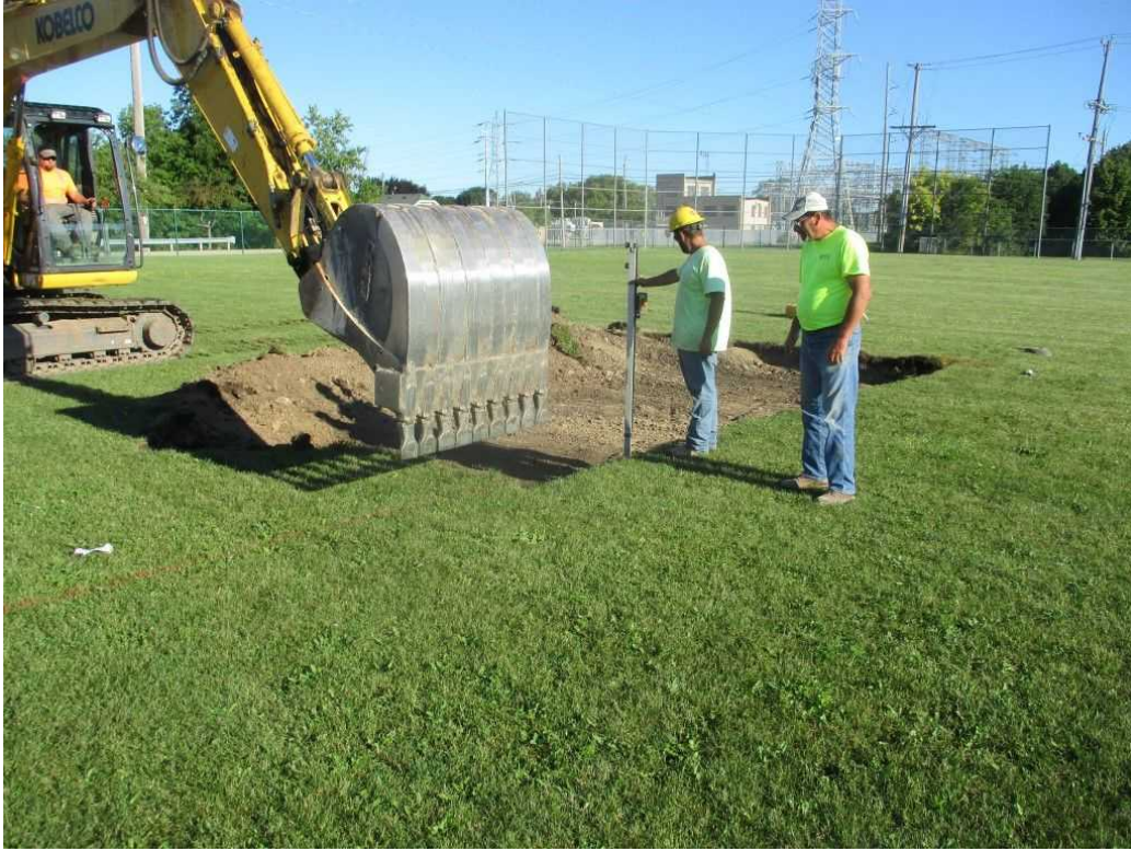
EXCAVATION FOR PLAYGROUND FOUNDATION, FACING NORTHWEST
