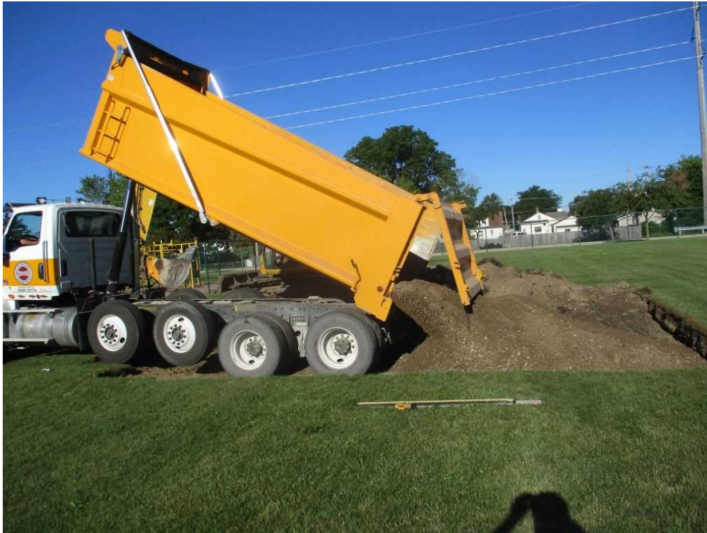
DELIVERY OF AGGREGATE BASE MATERIAL, FACING NORTH
