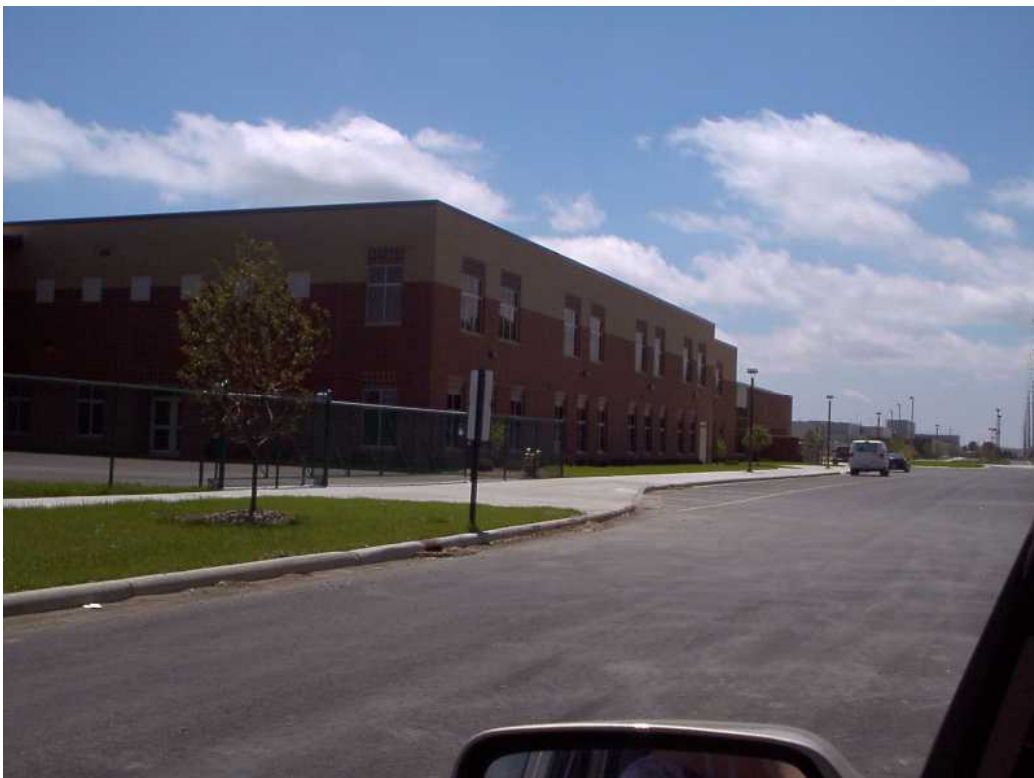
PAVED ACCESS DRIVE AND WALK, FACING SOUTHEAST
