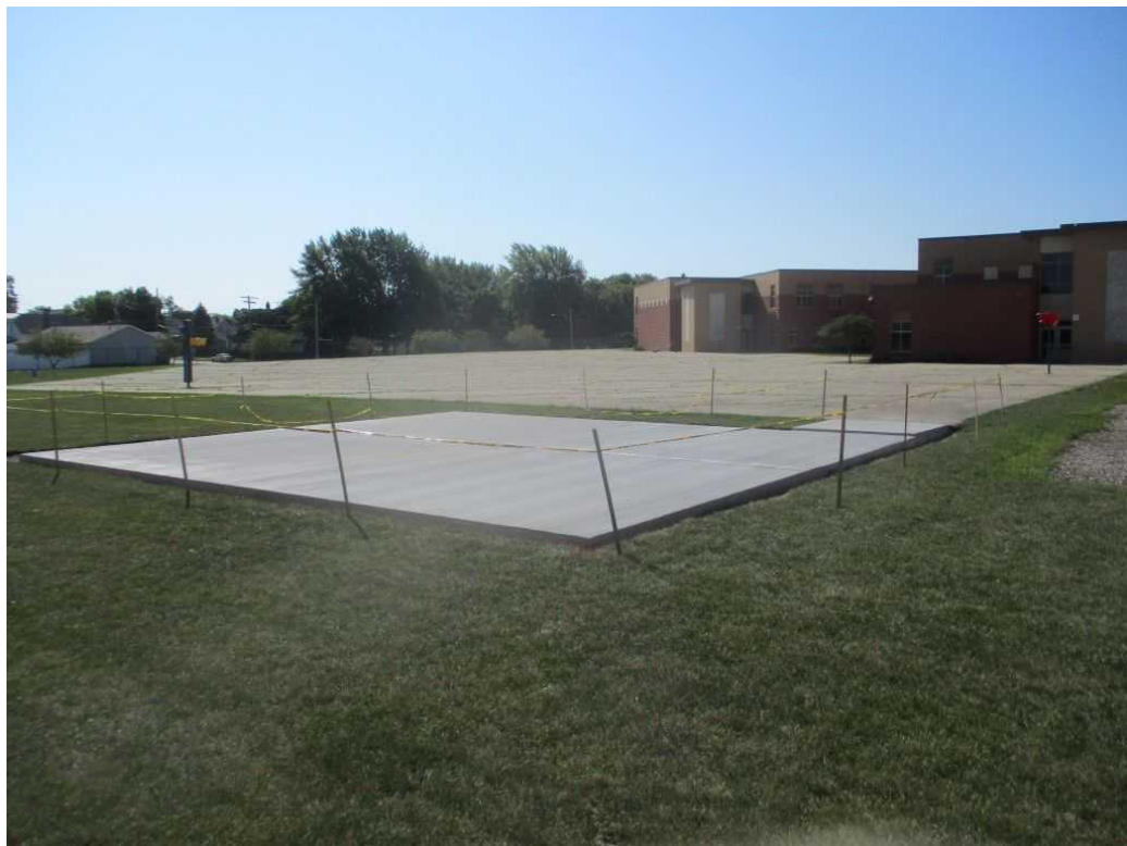
CONCRETE FOUNDATION SLAB, FACING SOUTHEAST
