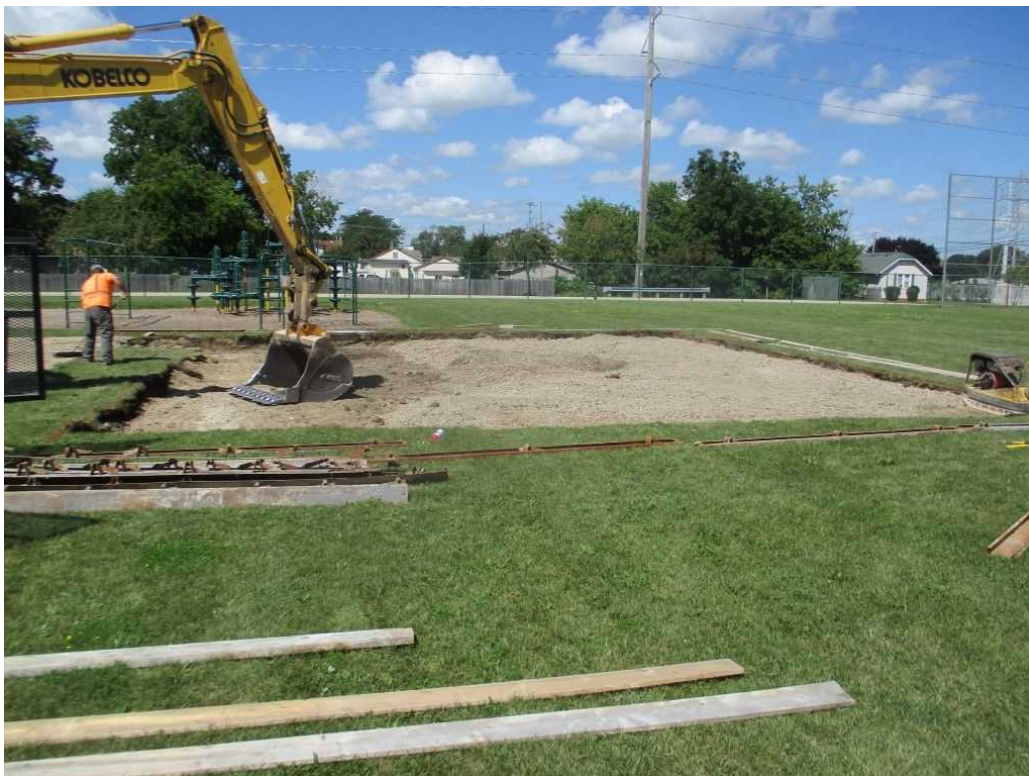
COMPACTION OF AGGREGATE BASE, FACING WEST
