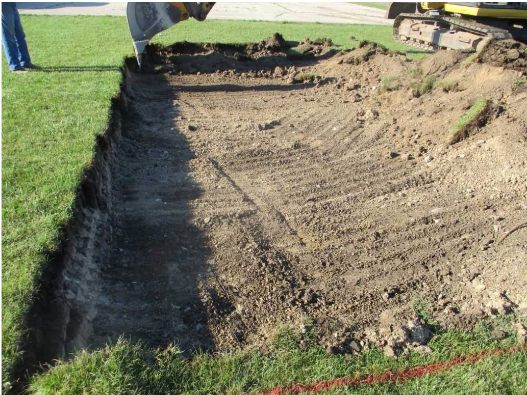
EXCAVATION FOR PLAYGROUND FOUNDATION, FACING SOUTH
