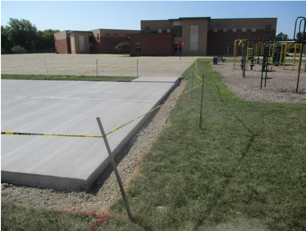
CONCRETE FOUNDATION SLAB, FACING SOUTH
