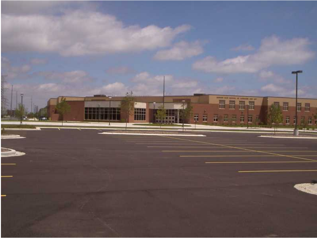
PAVED PARKING LOT AND FRONT ENTRANCE AREA, FACING NORTH
