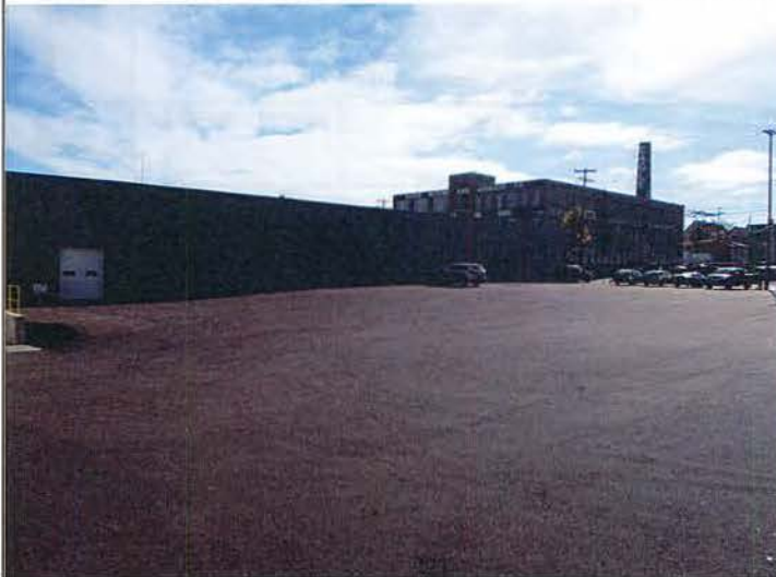
Title: Facing SE showing asphalt paved barrier replacing building D
