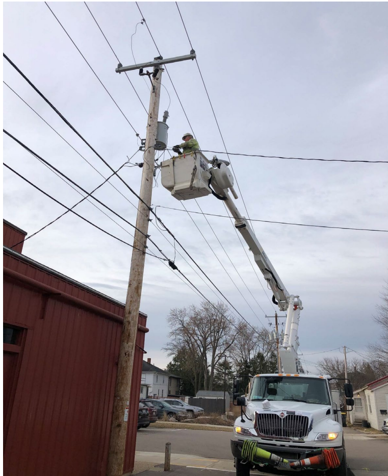
Electrical service line to the Nail Boutique being removed to allow the SVE wells along the south side of the building to be installed
