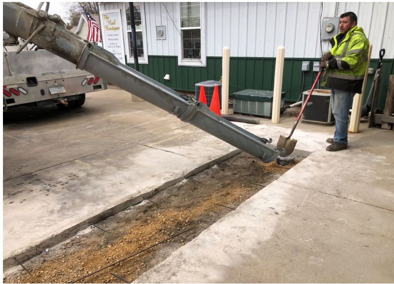
Concrete replacement along the front of the Nail Boutique
