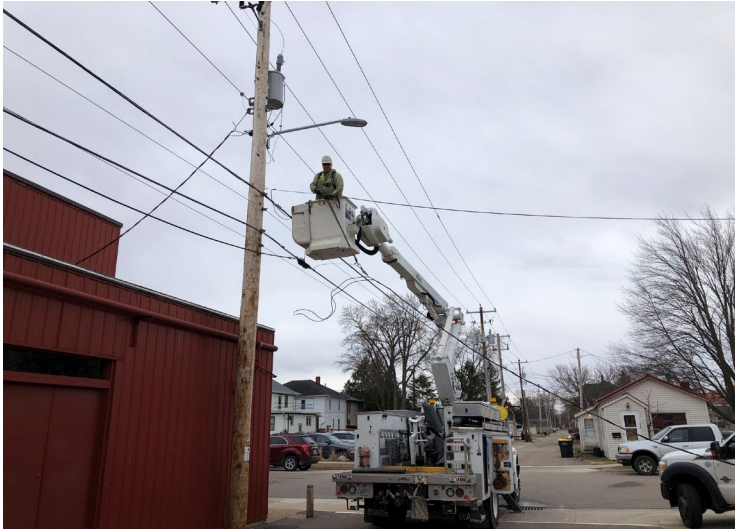
Re-energizing the Nail Boutique electrical power supply
