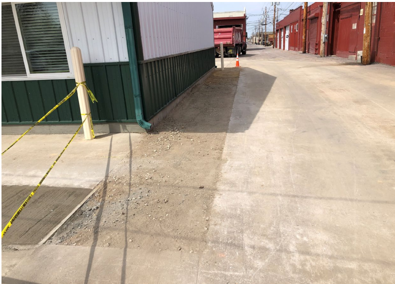
Temporary gravel surface cover until additional trenching work is completed
