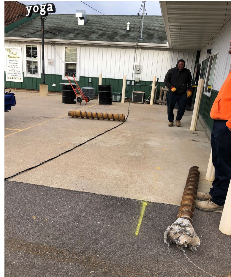
Electrical service line to the Nail Boutique being removed to allow the SVE wells along the south side of the building to be installed
