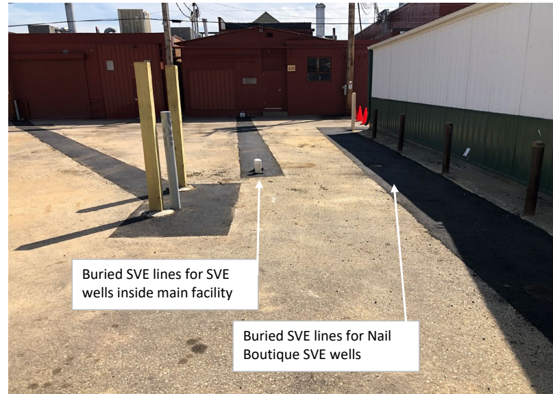
Completed trenches finished with asphalt surface cover
