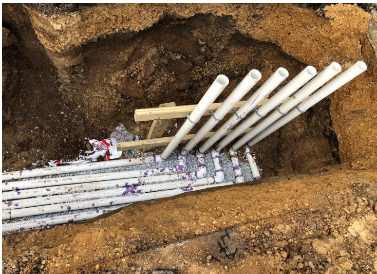
Underground SVE lines for the Nail Boutique SVE system being installed
