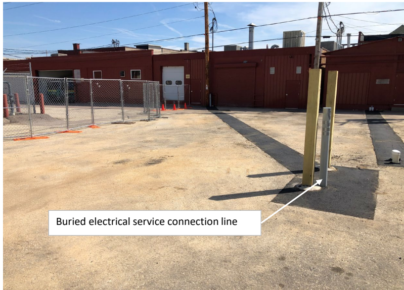
Buried electrical conduit awaiting electrical service connection
