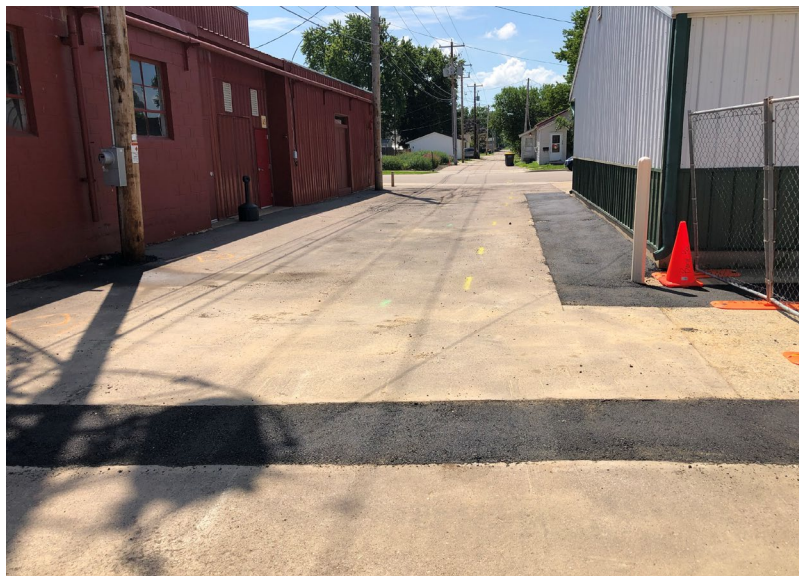
Buried electrical conduit awaiting electrical service connection
