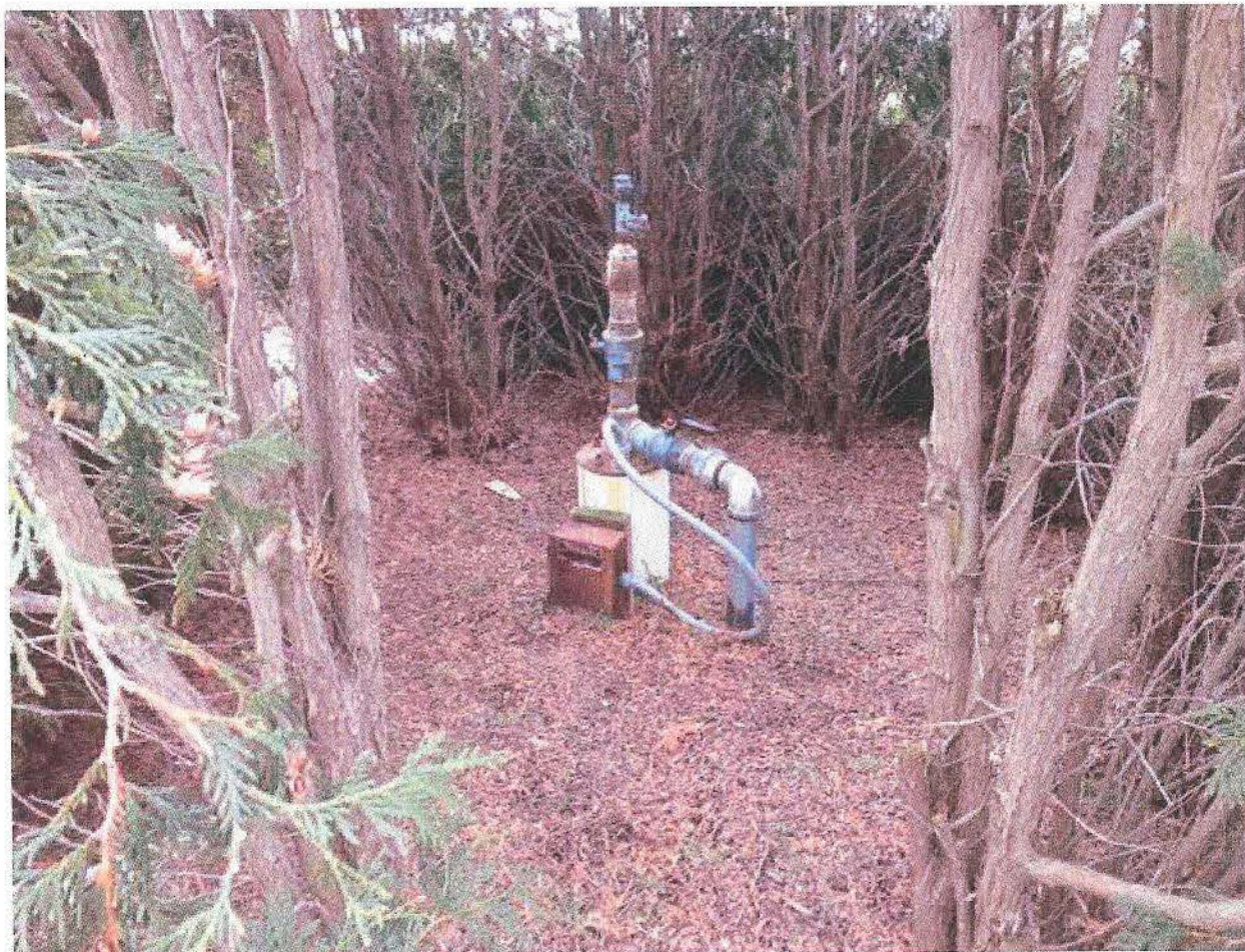
Photo 5 Groundwater Extraction Well
