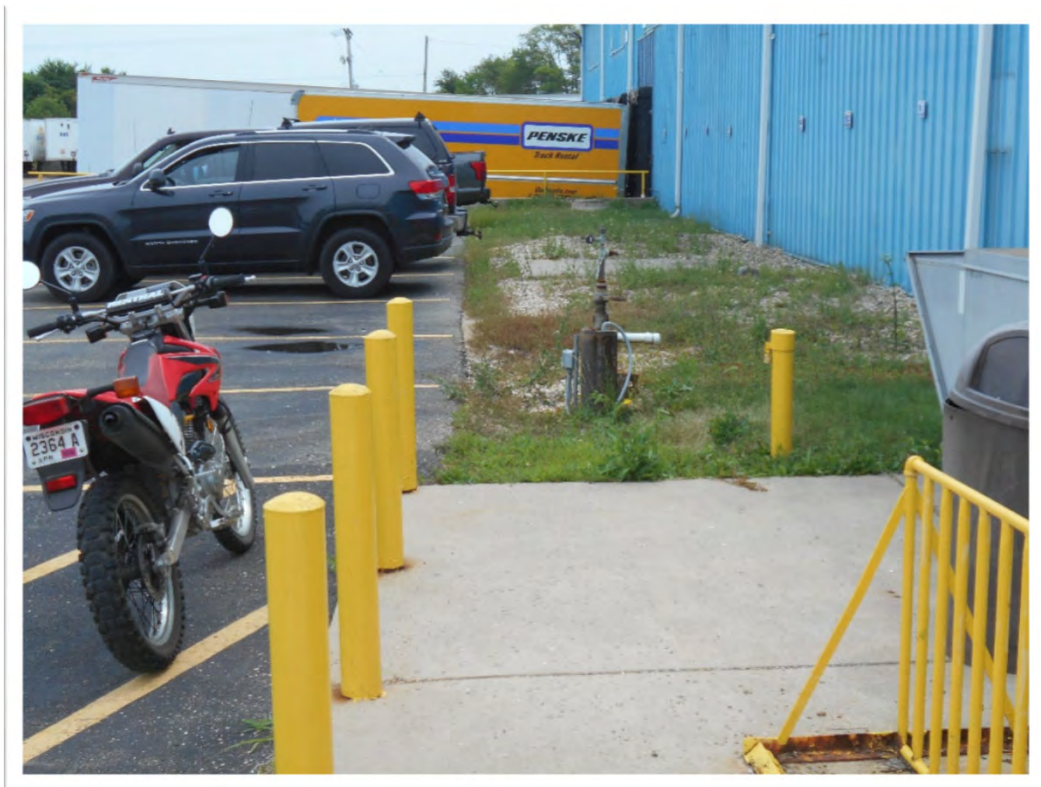
8.View looking east towards Extraction well EX-7R located on north side of Plant 2 in former sump source area.
