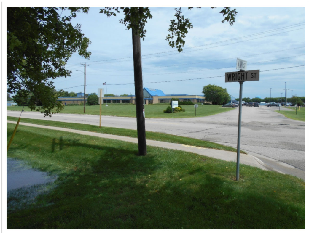
4. Looking east from west side of Wright Street towards main entrance to Plant 1.
