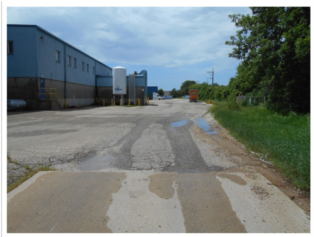
10. Looking west from north side of property. North wall of Plant 1 on left side of photo.
