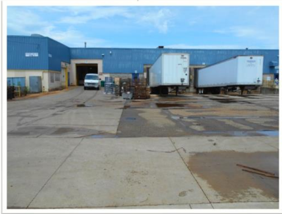
9. View looking north at loading docks on south side of Plant 1.
