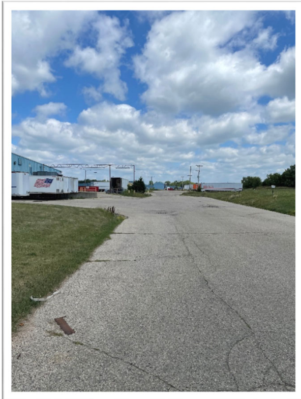
4.View looking north towards southeast half of east side of property.
