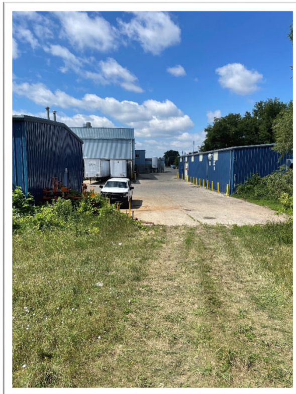
2. View looking northwest towards north side of property.
