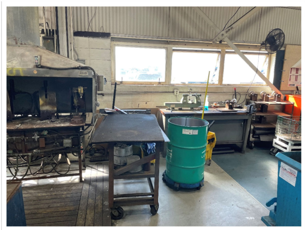
8. View looking south inside Plant 1 where low-level VOC's impacts occur in the sub-surface soil.
