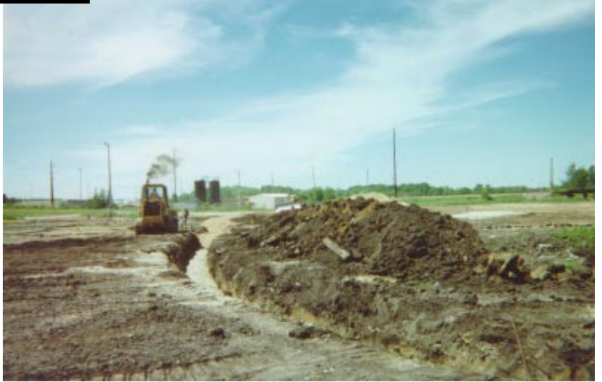
Installation of piping for Treatment Gates 1 and 2
