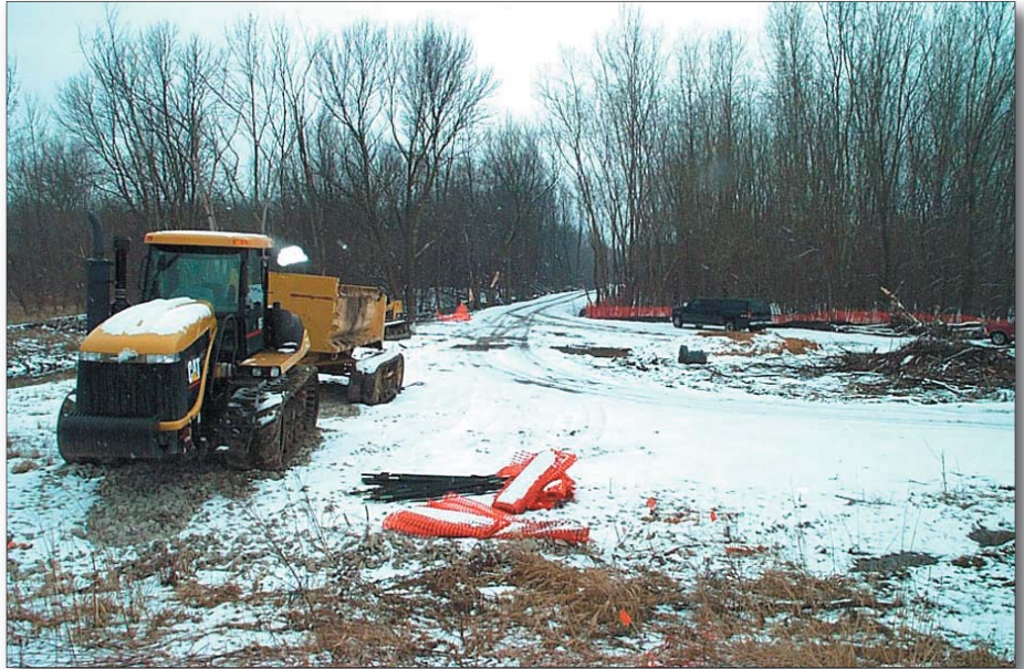
A bulldozer hauls soil from the new access road south of Bradley Road.
