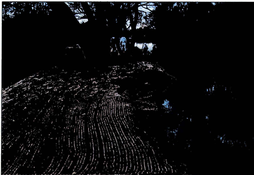
Photograph No.: 16 Photographer: Troy Thompson Date: 10/28/2009 Subject: Disturbed areas along the river banks were seeded and erosion control mats were placed along the banks. Hay mulch was placed on the upland areas.
