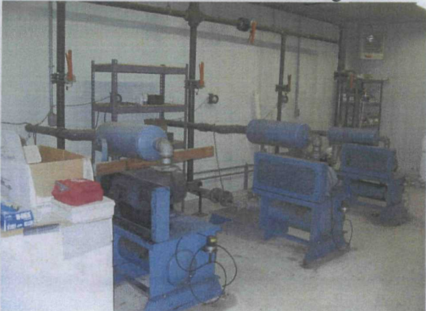
Inside view of GW Treatment building
