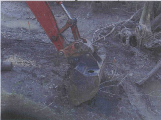
Sediment being excavated along Reach 4/5 of Little Menomonee River (August 31, 2009)
