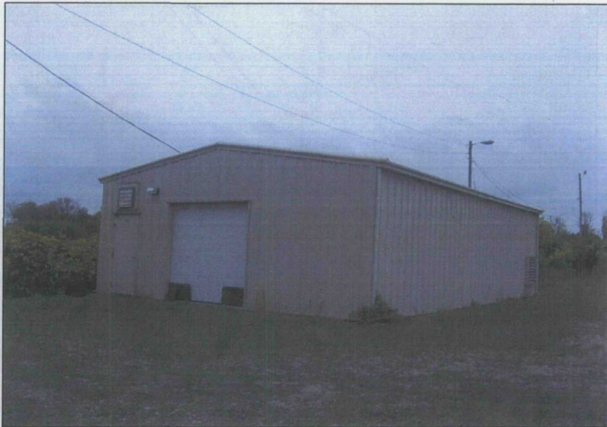
Photograph No.: 3 Photographer: Naren Babu Date: 10/09/2009 Subject: View of the groundwater treatment system building operated and maintained by Tronox.
