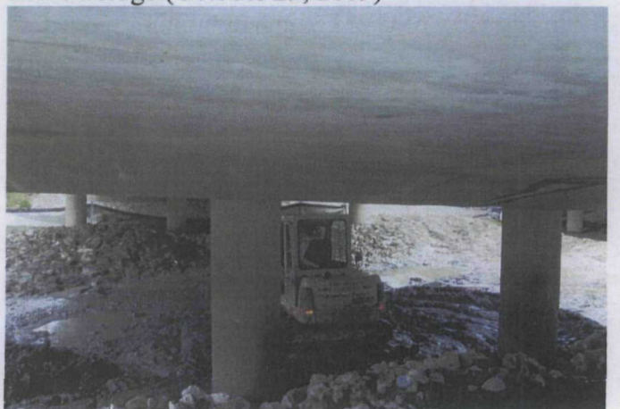
Sediment exaction work under Silver Spring Drive Bridge (October 29, 2009)
