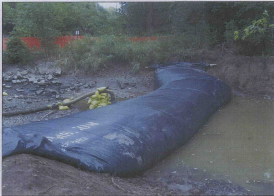
Photograph No.: 5 Photographer: Naren Babu Date: 08/25/2009 Subject: View of the water inflatable dam installed in the Little Menomonee River.
