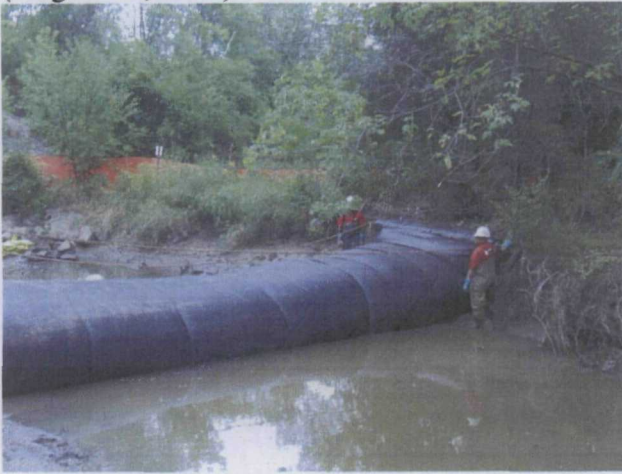
Dam installation prior to dredging river (August 29, 2009)
