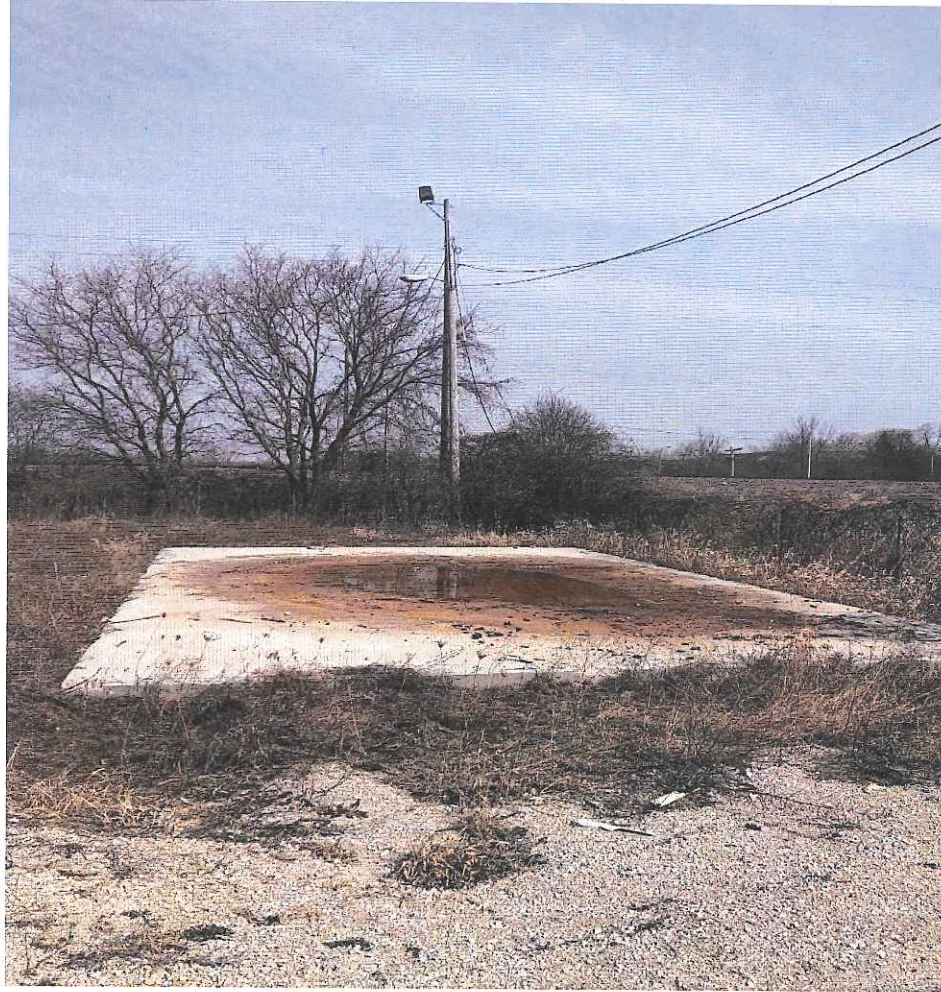
Concrete pad of former groundwater treatment building
