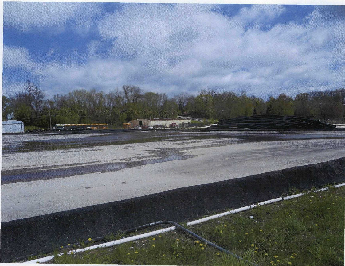
Dewatering pad at former Tecumseh property
