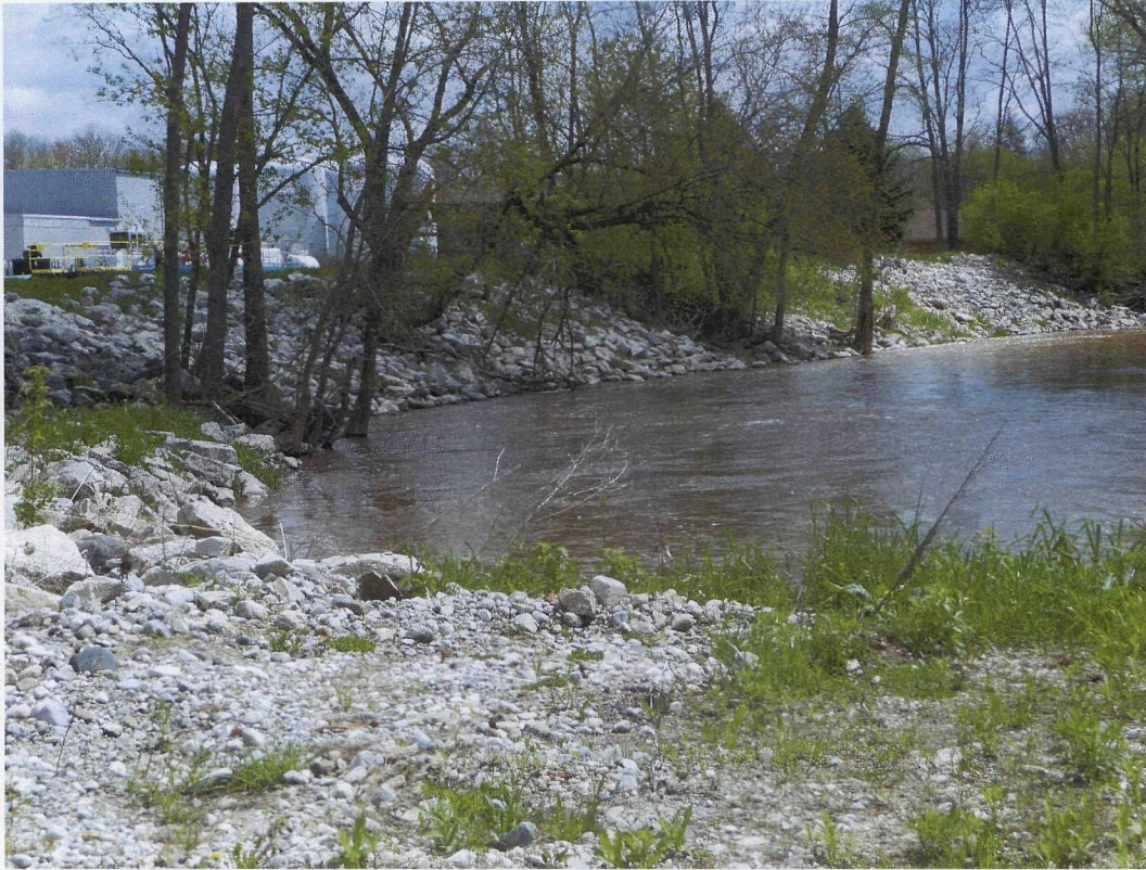
Upper River - restored river bank at Former Tecumseh Property (preferential pathway excavation)
