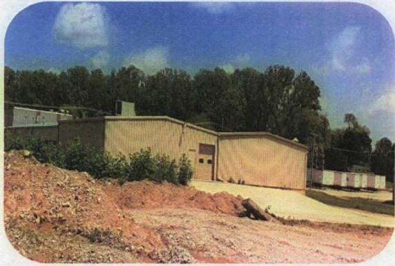
Drainage ditch grading in progress at Maryland avenue dewatering pad
