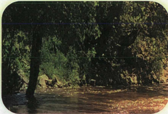
Rip rap placed at river shoreline at former Tecumseh plant location after excavation of armored areas
