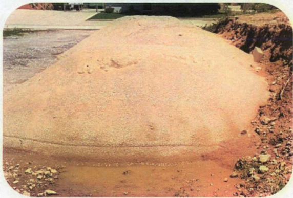
Sand at Maryland avenues dewatering pad
