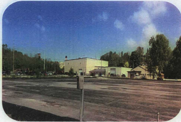
Dewatering pad at Former Tecumseh Plant
