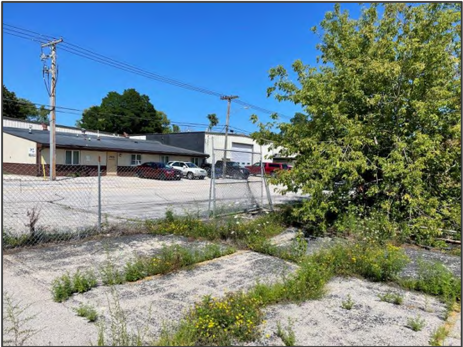
PHOTO NO. 10: View of fence along the north side of the Site.
