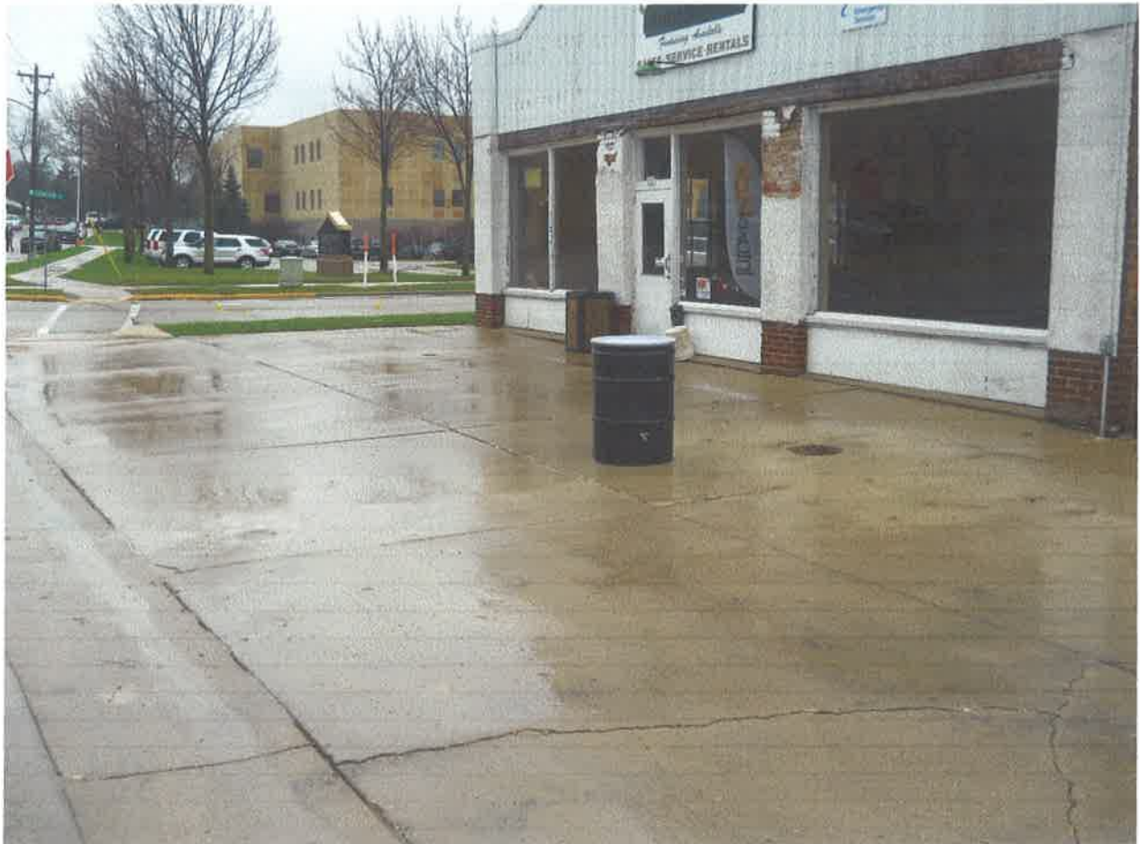
Photo #2: On site building looking southwest. (4/3/2017)
