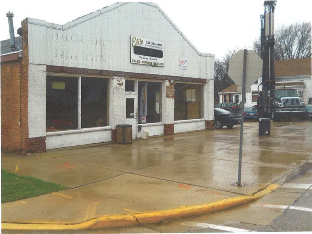
Photo #1: On site building looking northwest. (4/3/2017)
