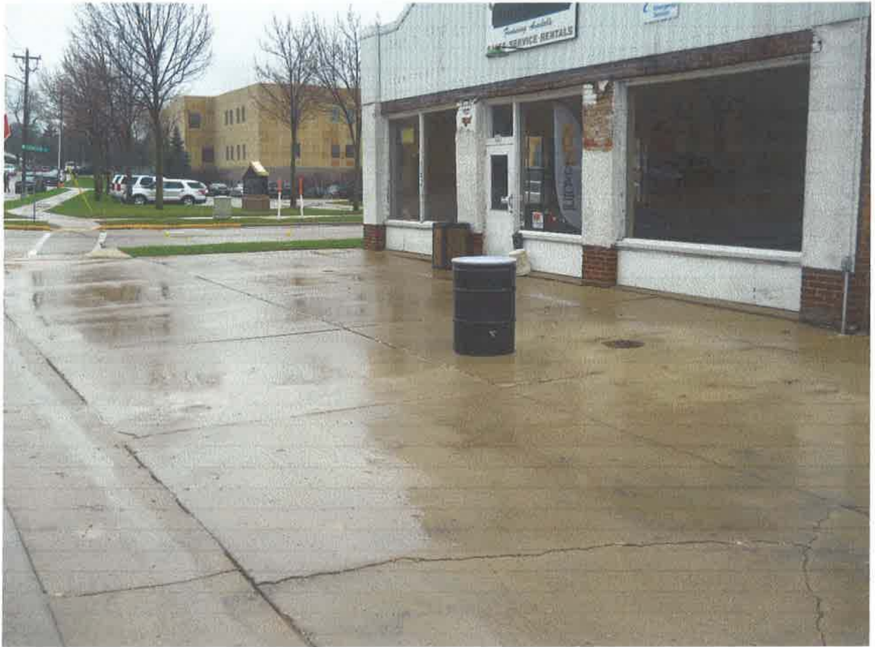
Photo #2: On site building looking southwest. (4/3/2017)
